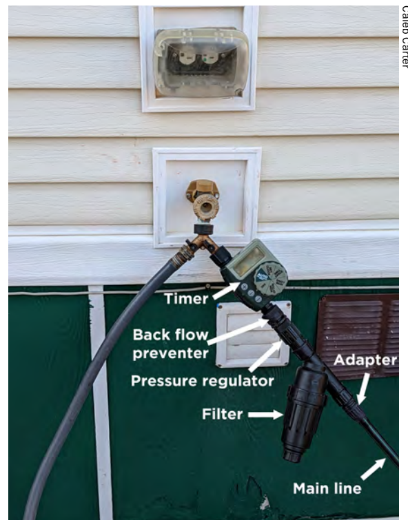
Typical drip system connection to a water source. Using a timer allows for automation and the hose splitter allows the use of a hose without disconnecting the drip system.
