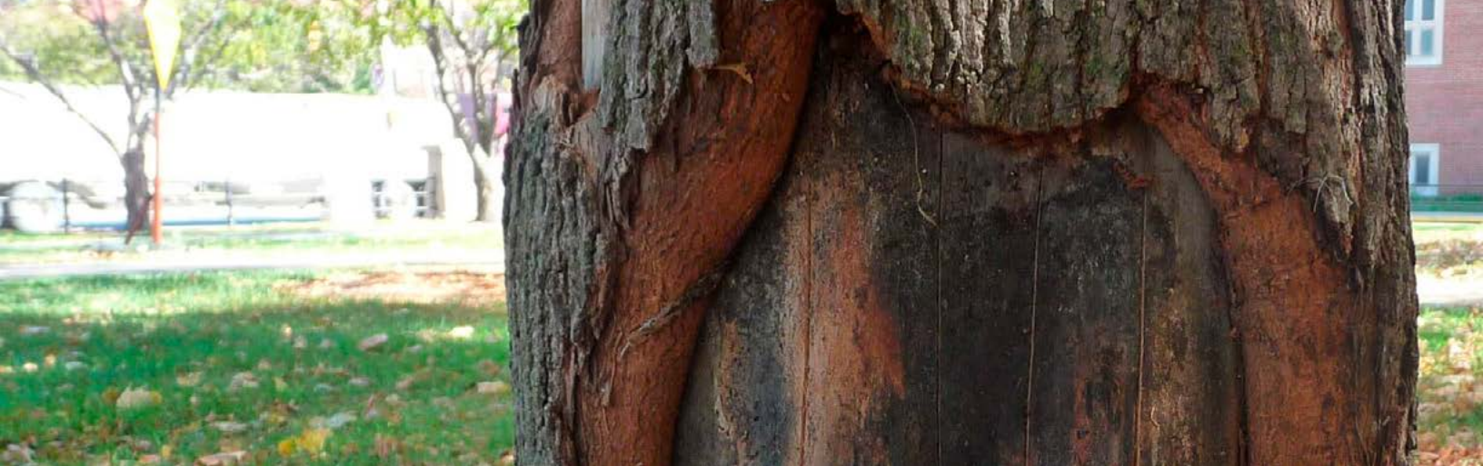
Tree trunk damaged by construction equipment developing wound wood around the edges to eventually seal the wound. Photo by Purdue Extension - Forestry and Natural Resources.
