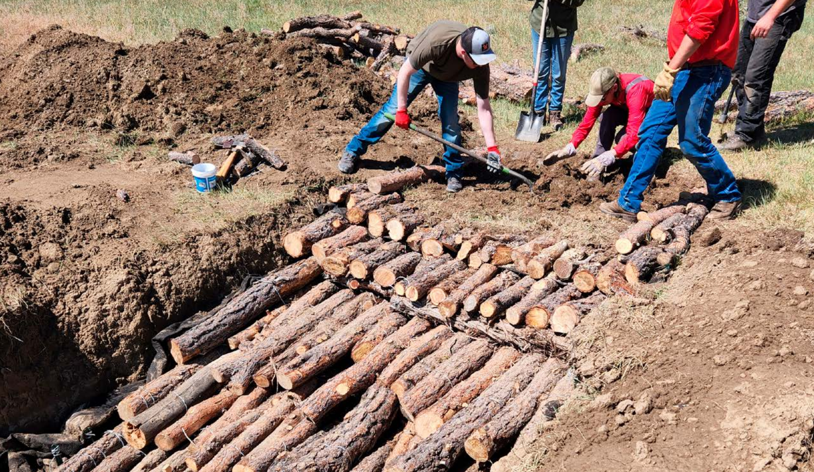
Log and fabric structure in northeastern Johnson County. Photo courtesy of Clear Creek Conservation District.
