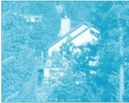
Combustible house with no defensible space
