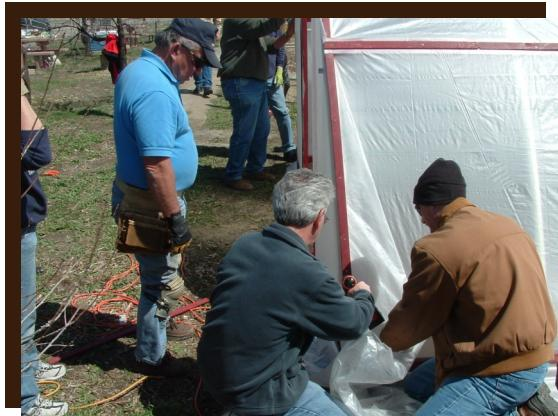
Keeping the plastic stretched, attach one side by sandwiching the plastic poly covering between a furring strip onto the baseboard, using a 1 in. deck screws, every 12 in.
