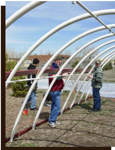
Mark the purlins every 36 in. where they will be attached to each 2 in. ribs. Two purlins will be attached 60 in. above the end of each pipe and one down the top middle of the hoop house. Marking the two end hoops and running a string can easily achieve a straight line.
