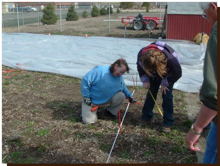
Along both lengths of the Hoop House and inside the string, drive 24 in. rebar stakes every 3 ft. apart, 12 in. deep, at 30 degree angles, until you reach the desired length.
