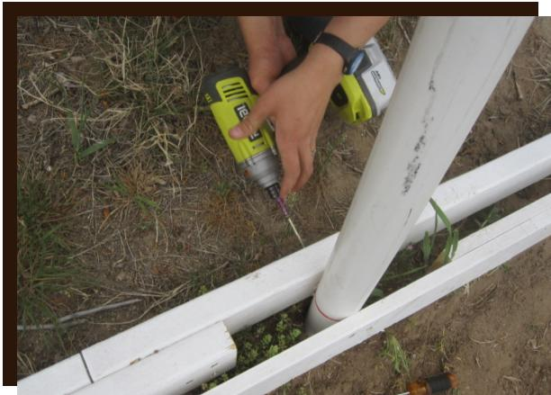
The outer baseboards should each be one 1 in. x 4 in. x 12 ft. and two 1 in. x 4 in. x 10 ft. boards, butted and fastened together by short (14 in.) brace pieces with the 12 ft. board in the middle. The inner baseboards should each be one 2 in. x 4 in. x 12 ft. and two 1 in. x 4 in. x 10 ft. Make sure the screws and brace pieces are facing toward the hoops when installing the baseboards.
