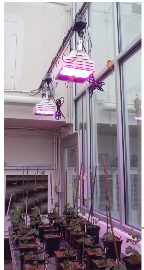
New high efficiency, low profile LED grow lights that have replaced the bulky high intensity lamps.
