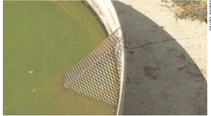
Escape ramp in water tank
