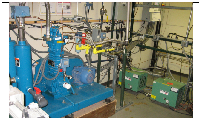
Figure 5. Low Pressure Compressor and Chillers
