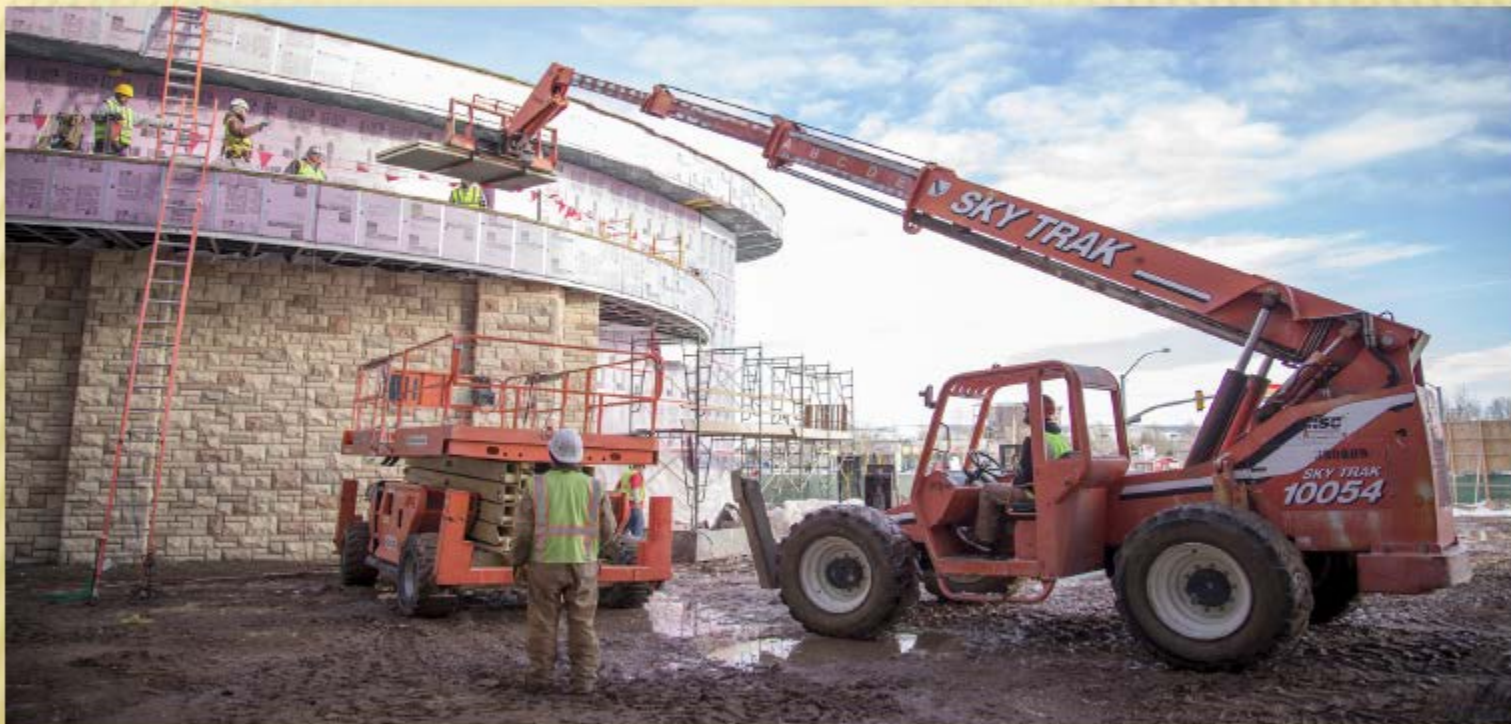
McMurry Foundation UW Legacy Hall
