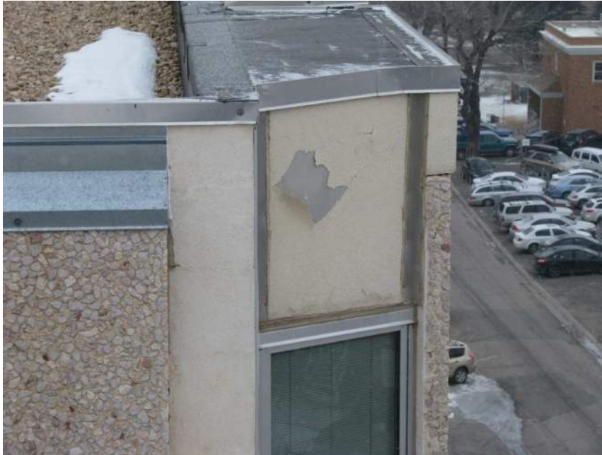
Photo 26 – Cracked Vertical Stucco Panels and Deteriorated Parapet Panel Coating at Orr Hall
