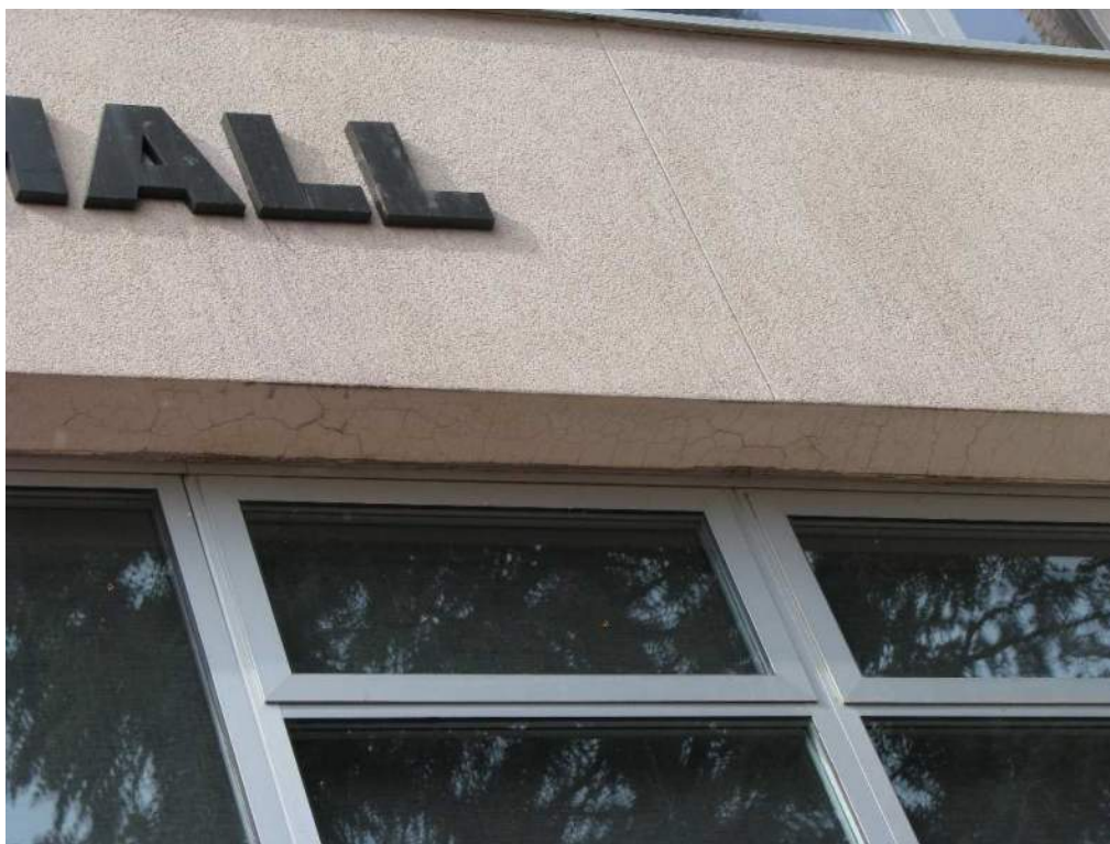
Photo 30 – Cracked Stucco Soffit at McIntyre Hall
