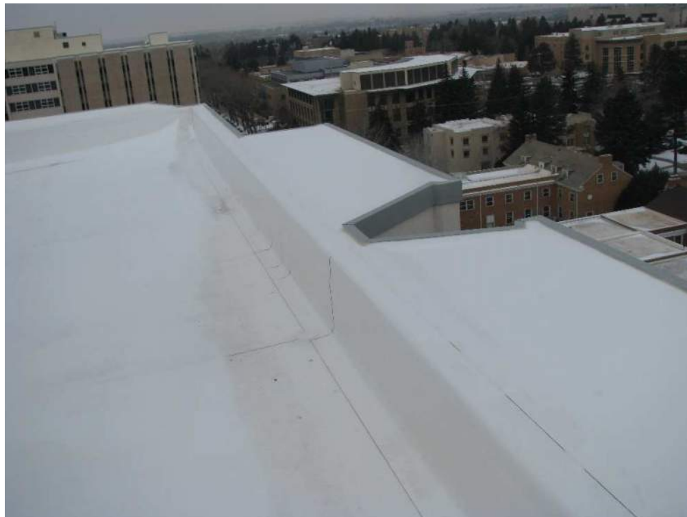
Photo 7 – New TPO Roofing at McIntyre Hall
