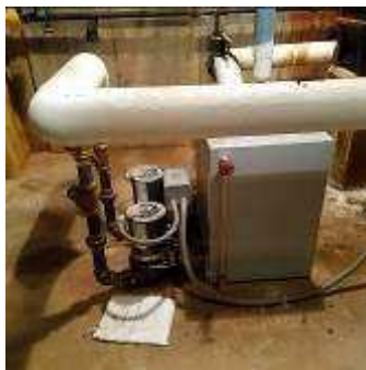
Figure 25: Hydronic Pumps
