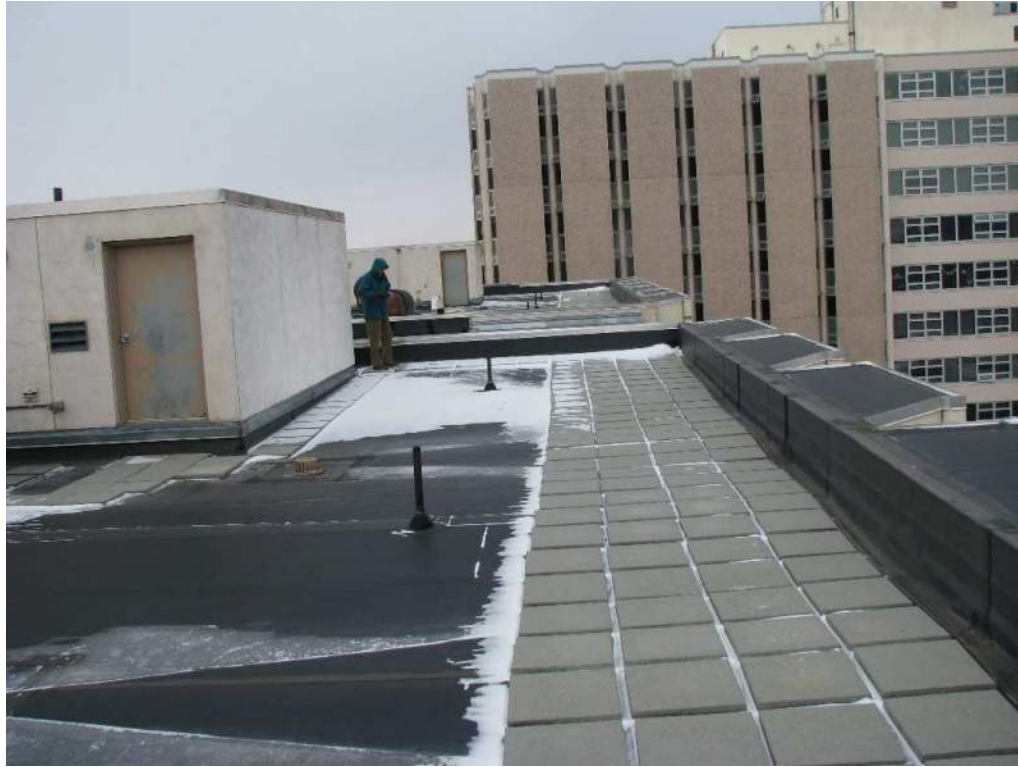
Photo 8 – New EPDM Roofing at Downey Hall
