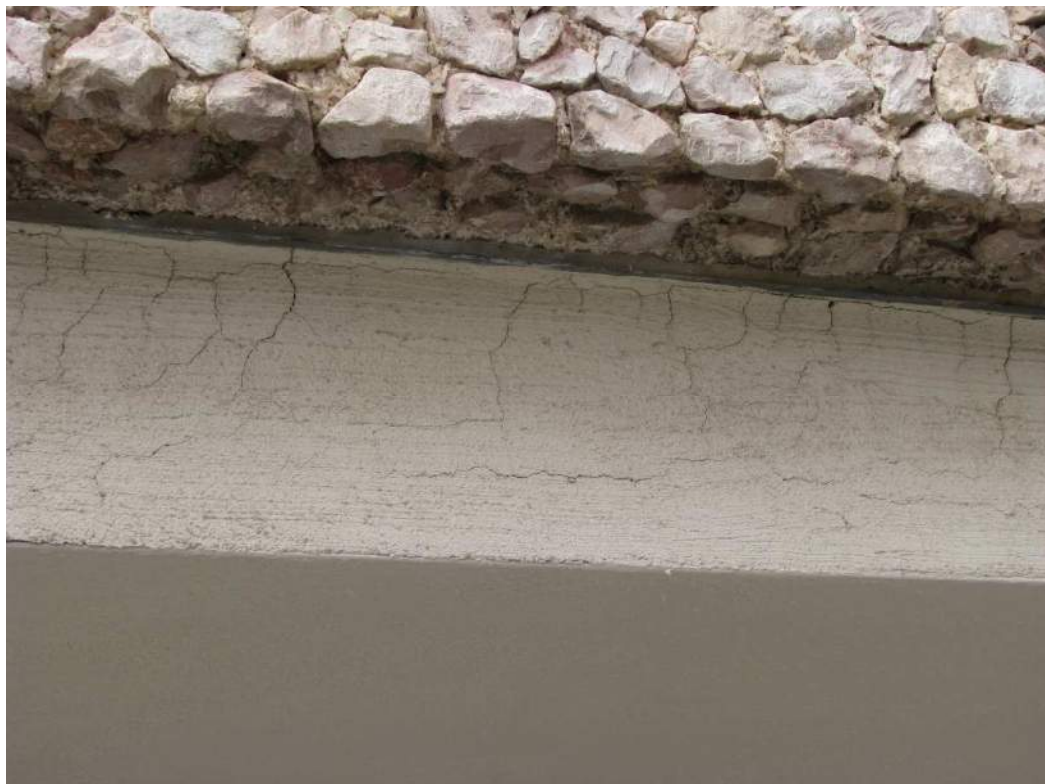
Photo 2 – Cracked Stucco Fascia Below Aggregate Panel at Downey Hall, Typical Elsewhere
