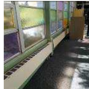
Figure 27: Corridor Radiation Heater
