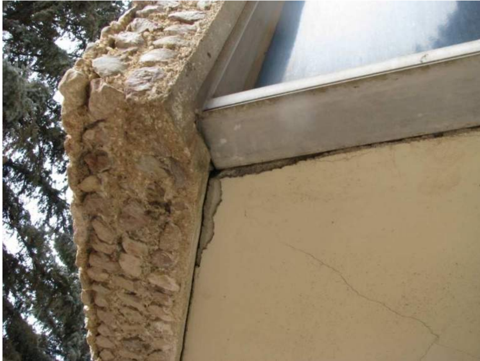
Photo 32 – Deteriorated Stucco Soffit at Downey Hall, Typical Elsewhere
