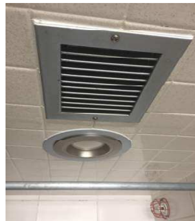
Figure 29: Typical Dorm Bathroom Exhaust Grille
