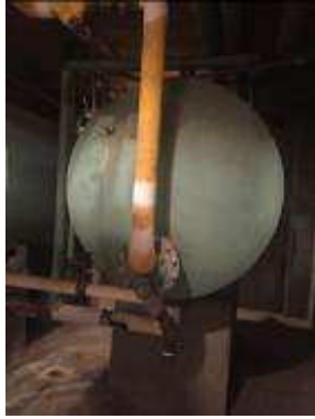
Figure 24: Steam Converter
