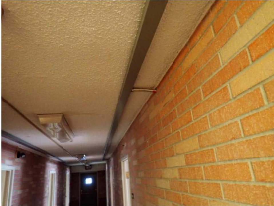
Photo 19 - Typical Data and Emergency Wiring Installation – Hill Hall
