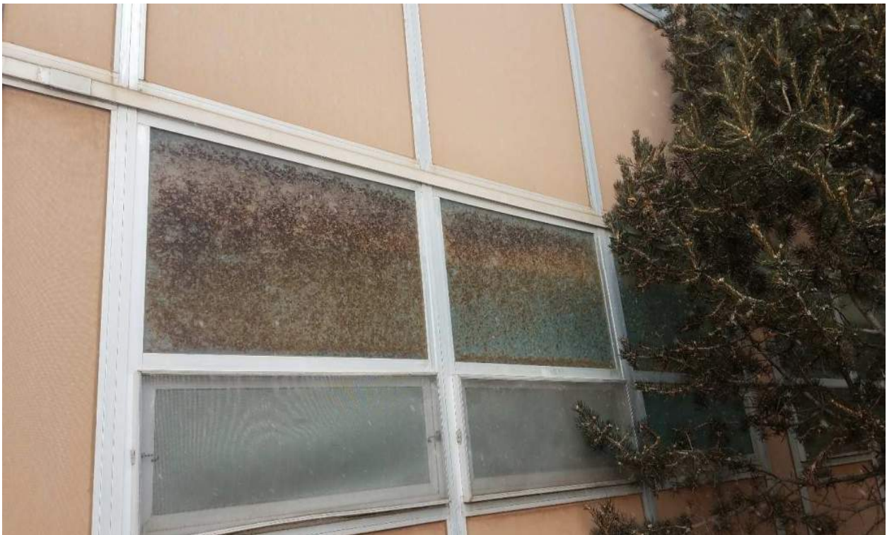
Photo 14 - Restroom Windows Showing Vinyl Obscuring Film Deteriorated by Sunlight at Crane Hall
