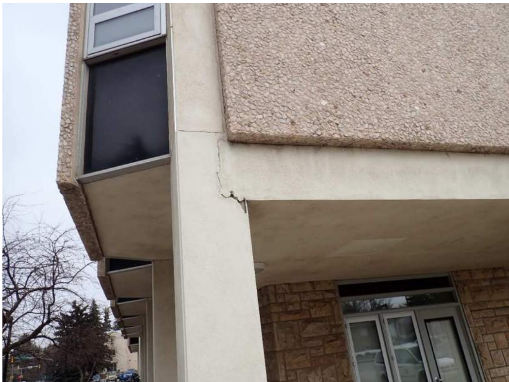
Photo 1 - Typical Structure at White Hall with Cracked Stucco
