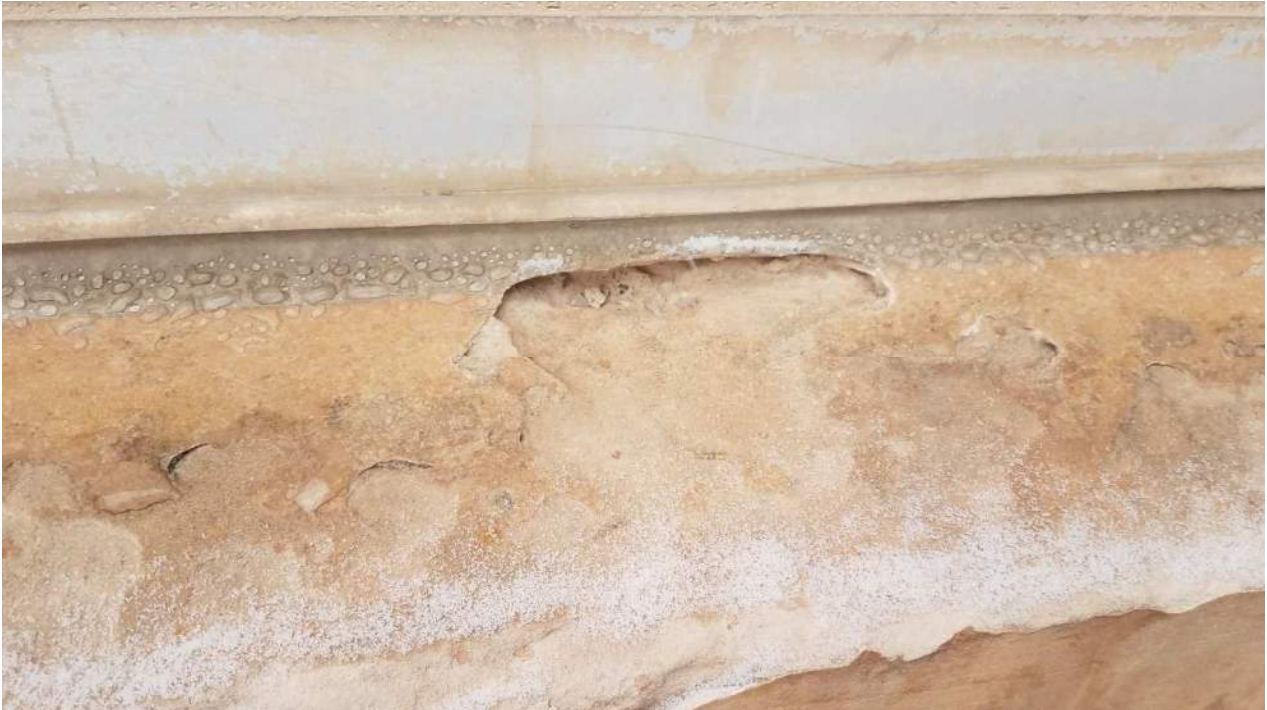
Photo 13 - Sandstone Foundation Erosion at Crane Hall
