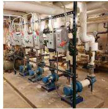
Figure 2: Hydronic Pumps
