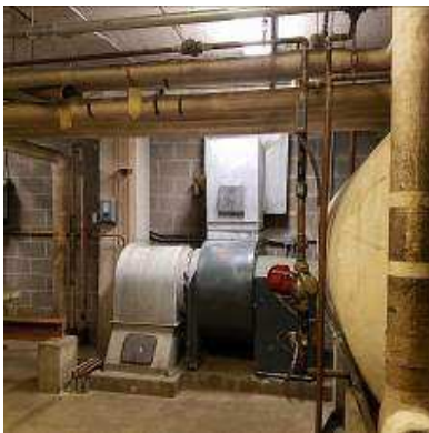
Figure 5: Exhaust Fan
