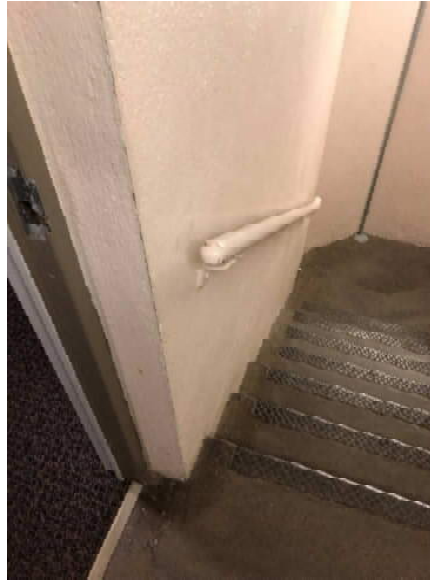
Figure 6: Missing handrail extensions at stairs
