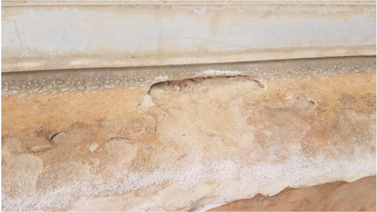
Photo 13 - Sandstone Foundation Erosion at Crane Hall
