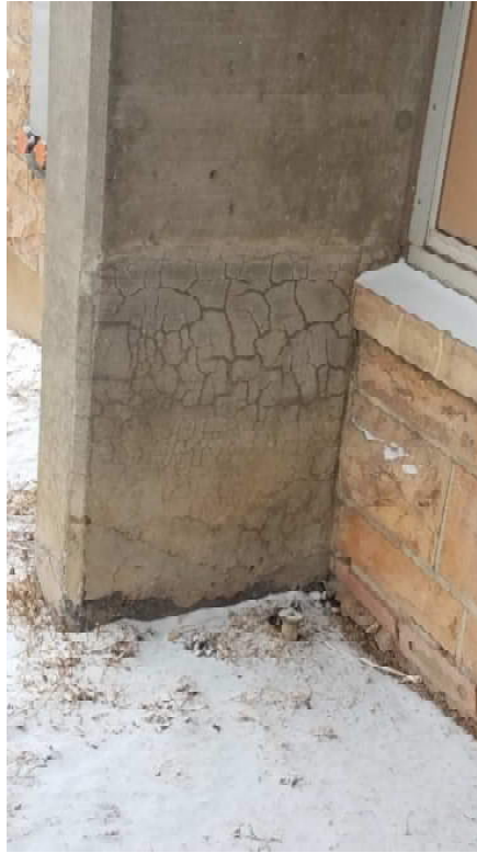
Photo 11 – Checked Concrete Column Surface at Crane Hall
