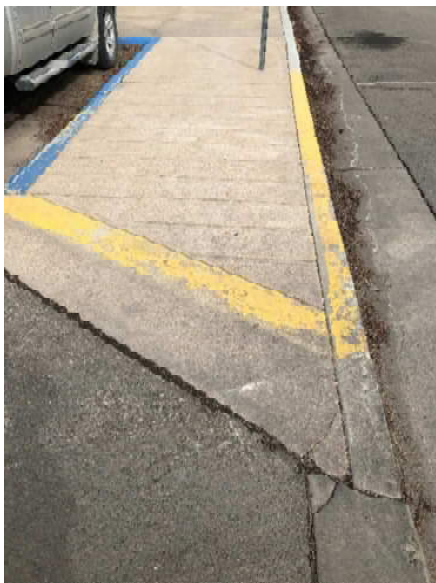
Figure 1: Sidewalk cracks in accessible route
