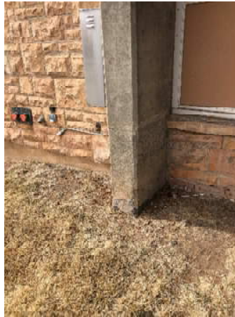
Figure 2 Exposed Concrete Fin
