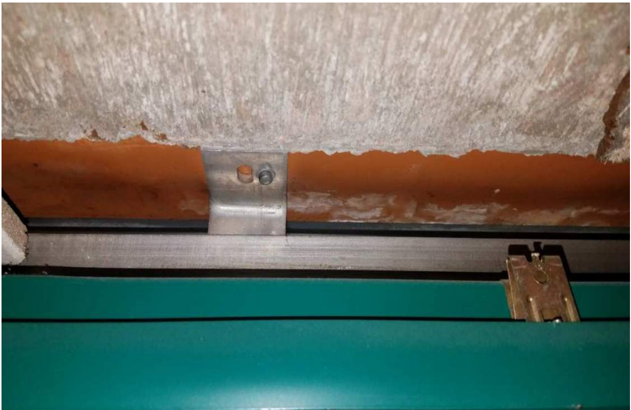
Photo 16 - Window Wall at Hill Hall Dormitory – No Insulation at Ceiling or Floor
