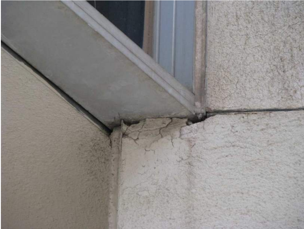
Photo 29 – Deteriorating Stucco Under Window Sill at McIntyre Hall
