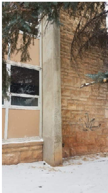
Photo 12 – Checked Concrete Column Surface at Crane Hall
