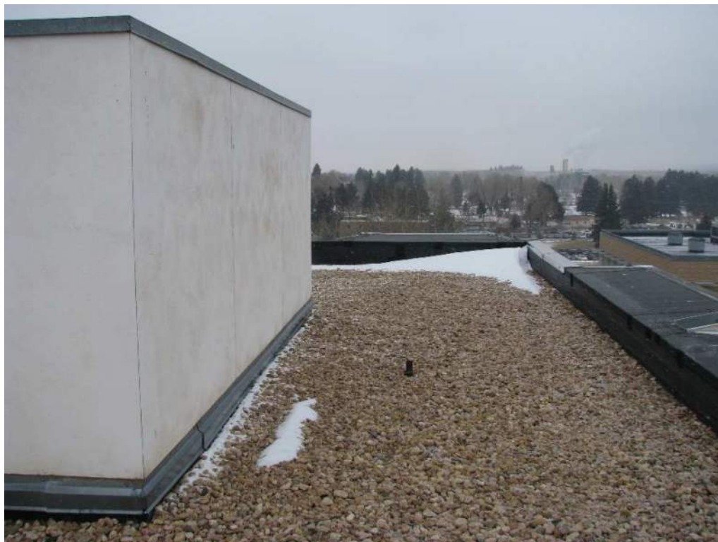
Photo 9 – Newer Ballasted EPDM Roofing at Orr Hall
