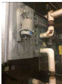
Figure 7: Fan Coil Unit
