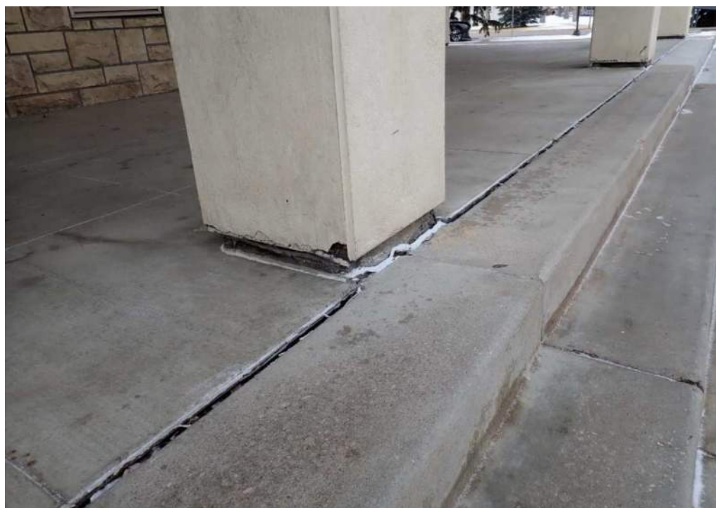
Photo 21 – Concrete Walk and Steps Separation at White Hall
