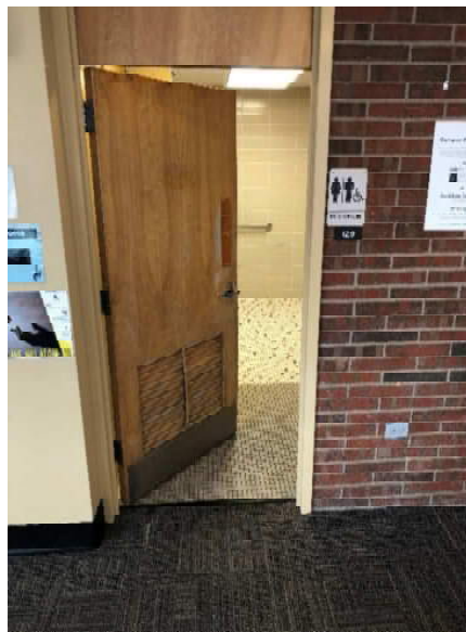
Figure 2: Door doesn't open a full 90 degrees
