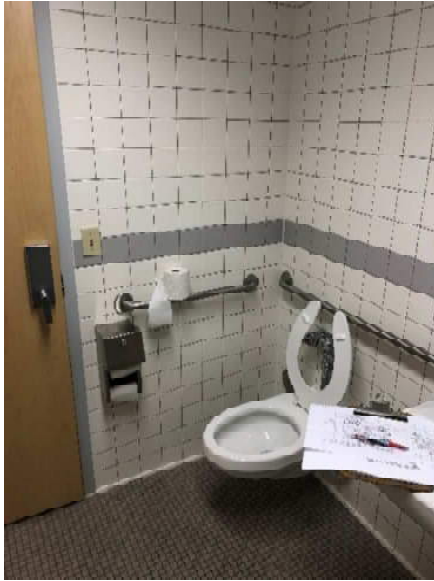
Figure 5: Toilet paper holder in 18" clear space And missing vertical grab bar
