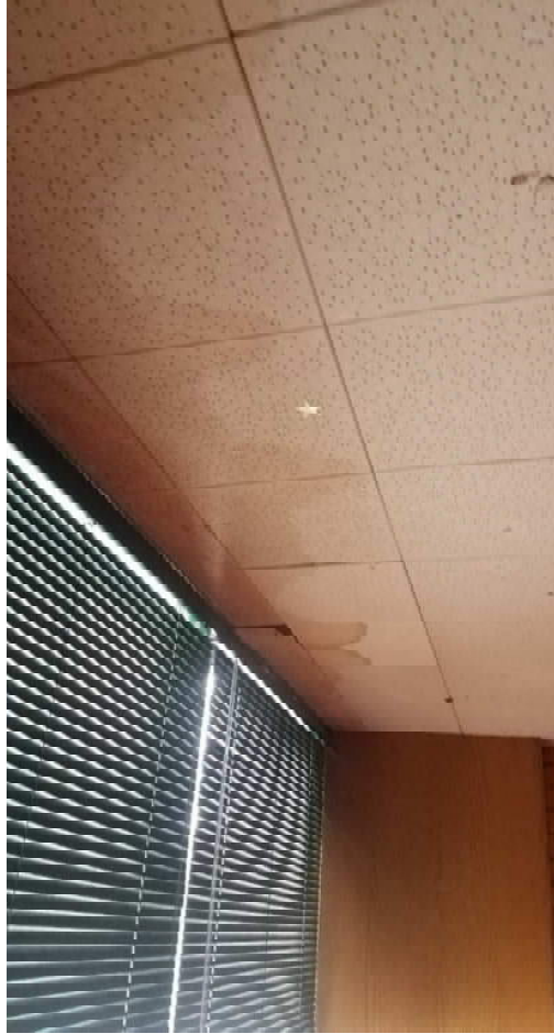
Photo 36 - Moisture Stains at Ceiling Tiles – Hill Hall
