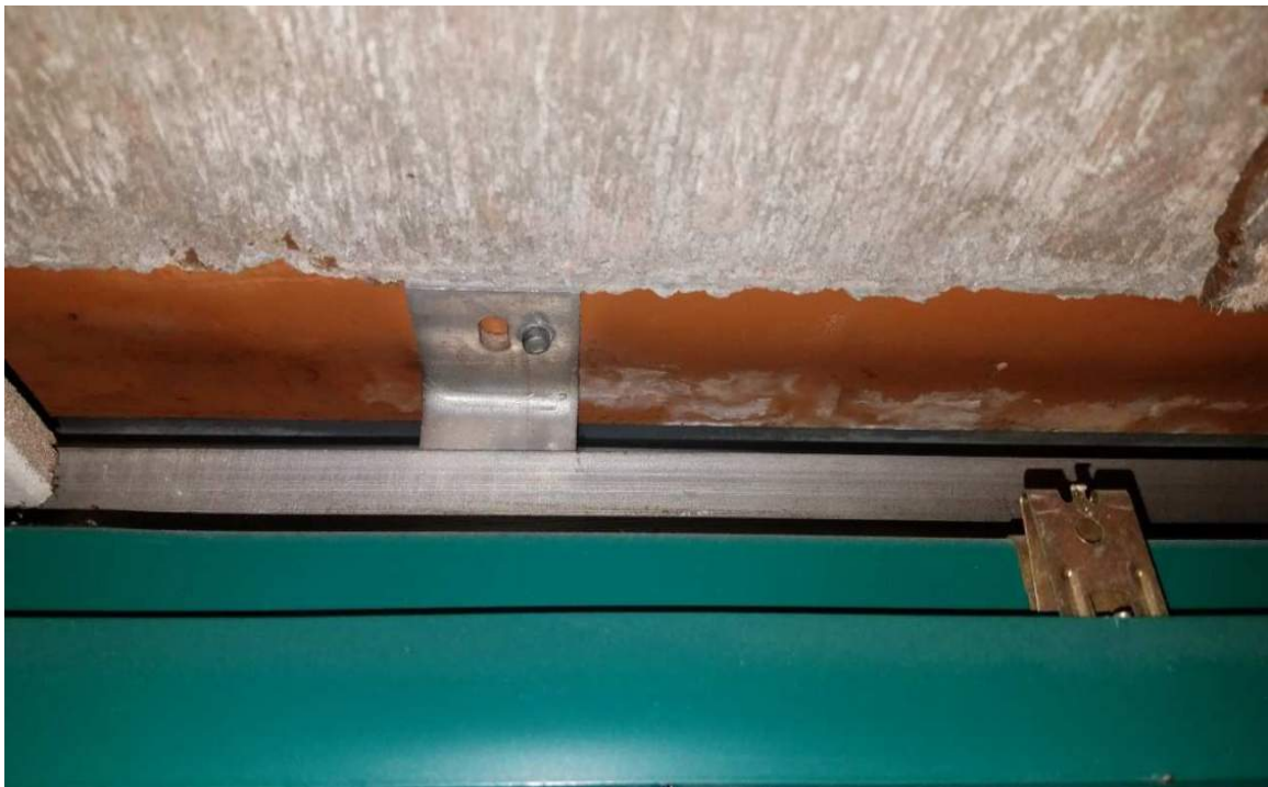
Photo 16 - Window Wall at Hill Hall Dormitory – No Insulation at Ceiling or Floor
