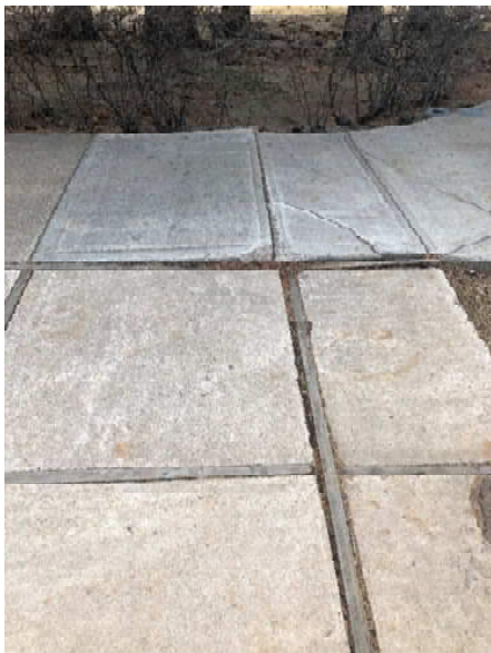
Figure 1: Sidewalk cracks in accessible route
