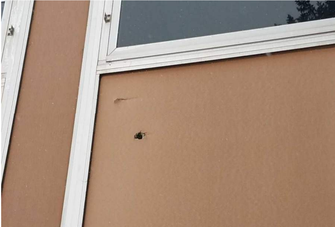
Photo 35 – Typical Damaged Panel at Crane Hall
