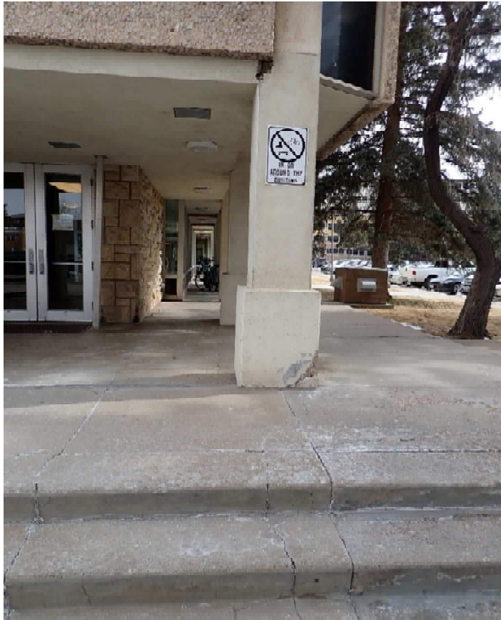
Photo 27 – Corner Column Cover and Head Stucco Cover Deterioration at Orr Hall
