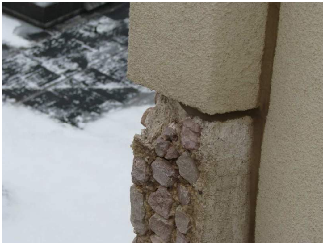
Photo 5 – Missing Stone Pieces in Aggregate Panel at Downey, Typical Elsewhere
