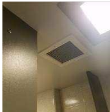
Figure 6: Typical Dorm Bathroom Exhaust Grille
