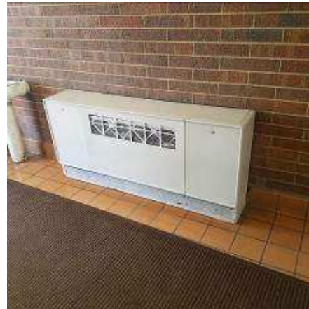
Figure 10: Hydronic Cabinet Unit Heater
