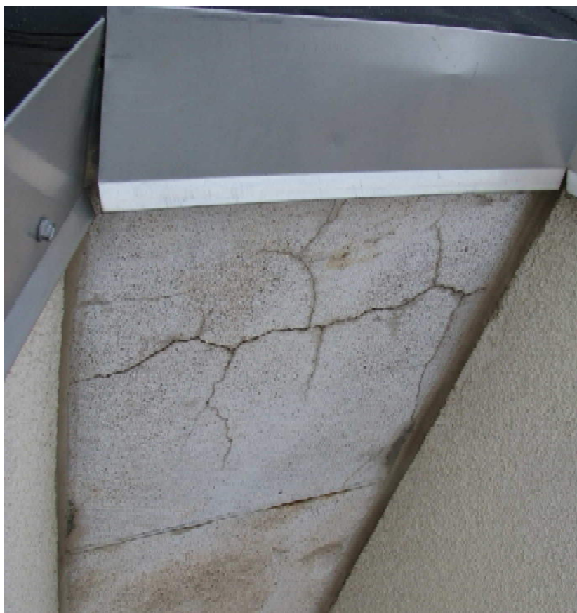
Photo 25 – Cracks in Vertical Stucco Fascia Strip at Downey Hall Typical All Washakie Dormitories
