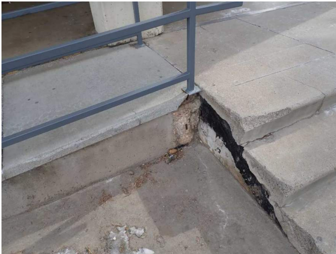
Photo 22 – Concrete Ramp and Stair Deterioration at Orr Hall
