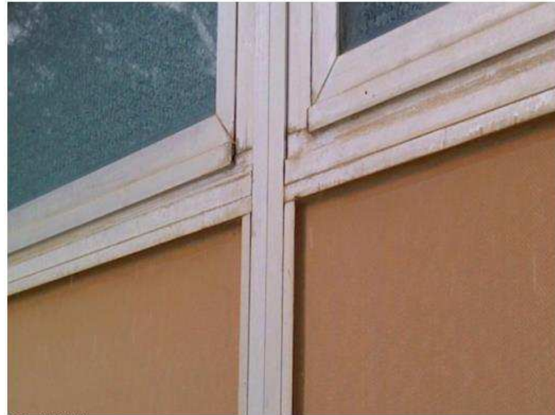
37 – Thermal Bridging through Curtainwall Framing Crane Hall
