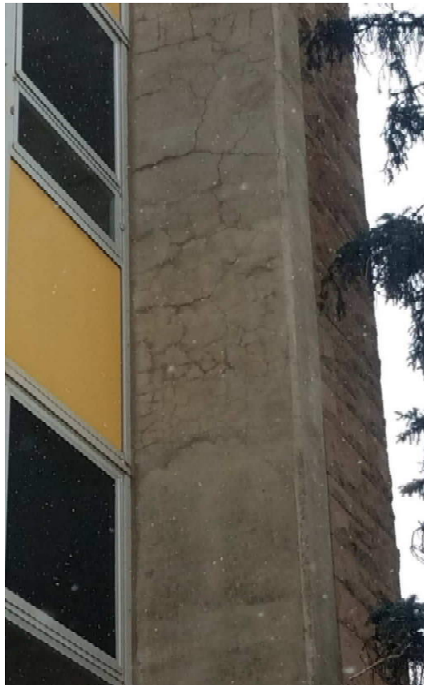
Photo 10 - Surface Checking at Architectural Concrete Column, Crane and Hill Halls
