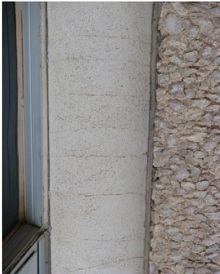
Photo 3 – Cracked Vertical Stucco Fascia at McIntyre Hall
