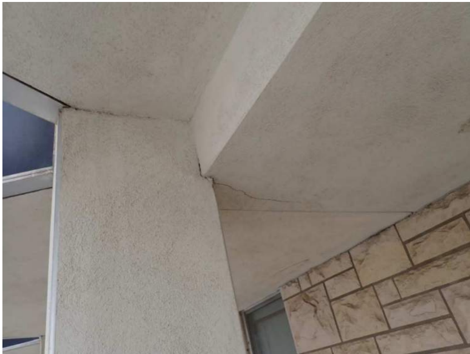
Photo 33 – Cracked Stucco Soffit Above Sidewalk at Orr Hall, Typical Elsewhere
