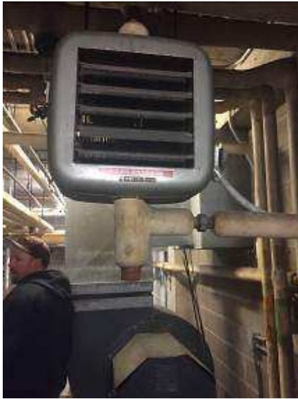
Figure 9: Hydronic Unit Heater
