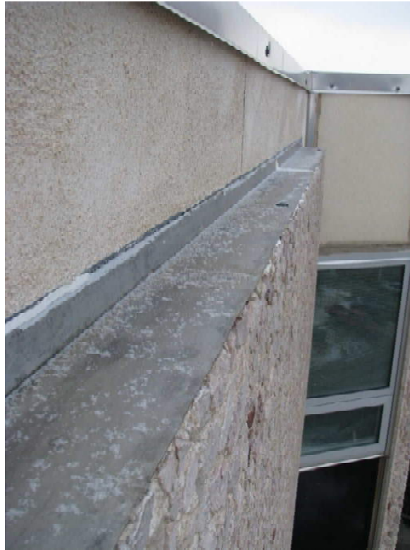
Photo 4 – Flashing at top of Precast Aggregate Panel, with extended parapet above at Downey Hall and at Orr Hall
