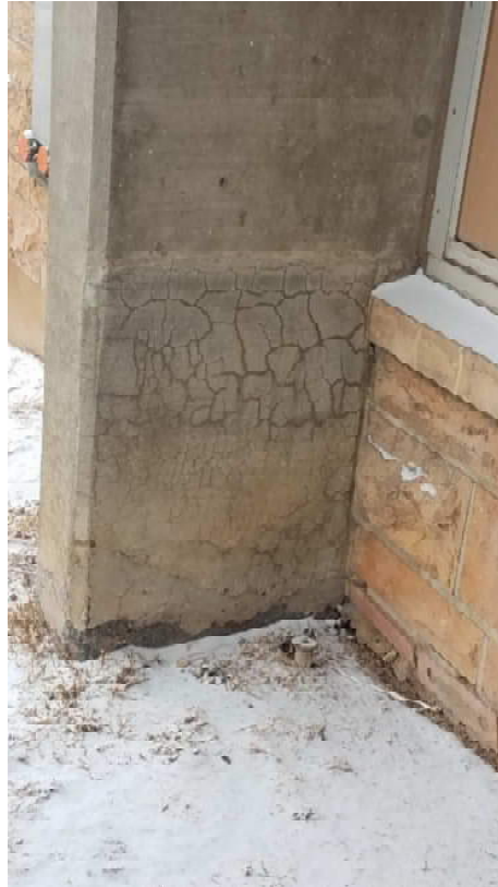
Photo 11 – Checked Concrete Column Surface at Crane Hall
