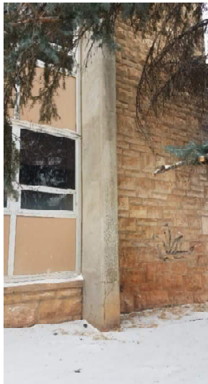
Photo 12 – Checked Concrete Column Surface at Crane Hall
