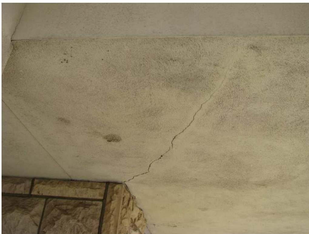
Photo 31 – Cracked Stucco Soffit, Ground Level, at McIntyre Hall
