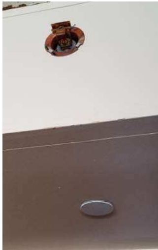
Figure 35: Within Units (typical) upper head missing cover
