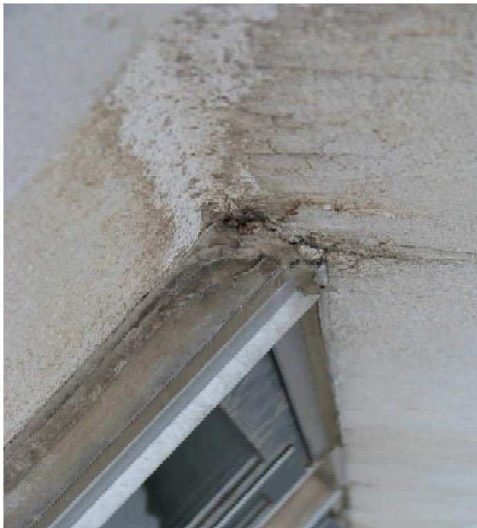
Photo 28 – Weathered Caulking at Window Head at McIntyre Hall
