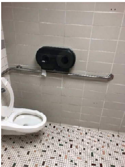
Figure 3: Missing vertical grab bar
