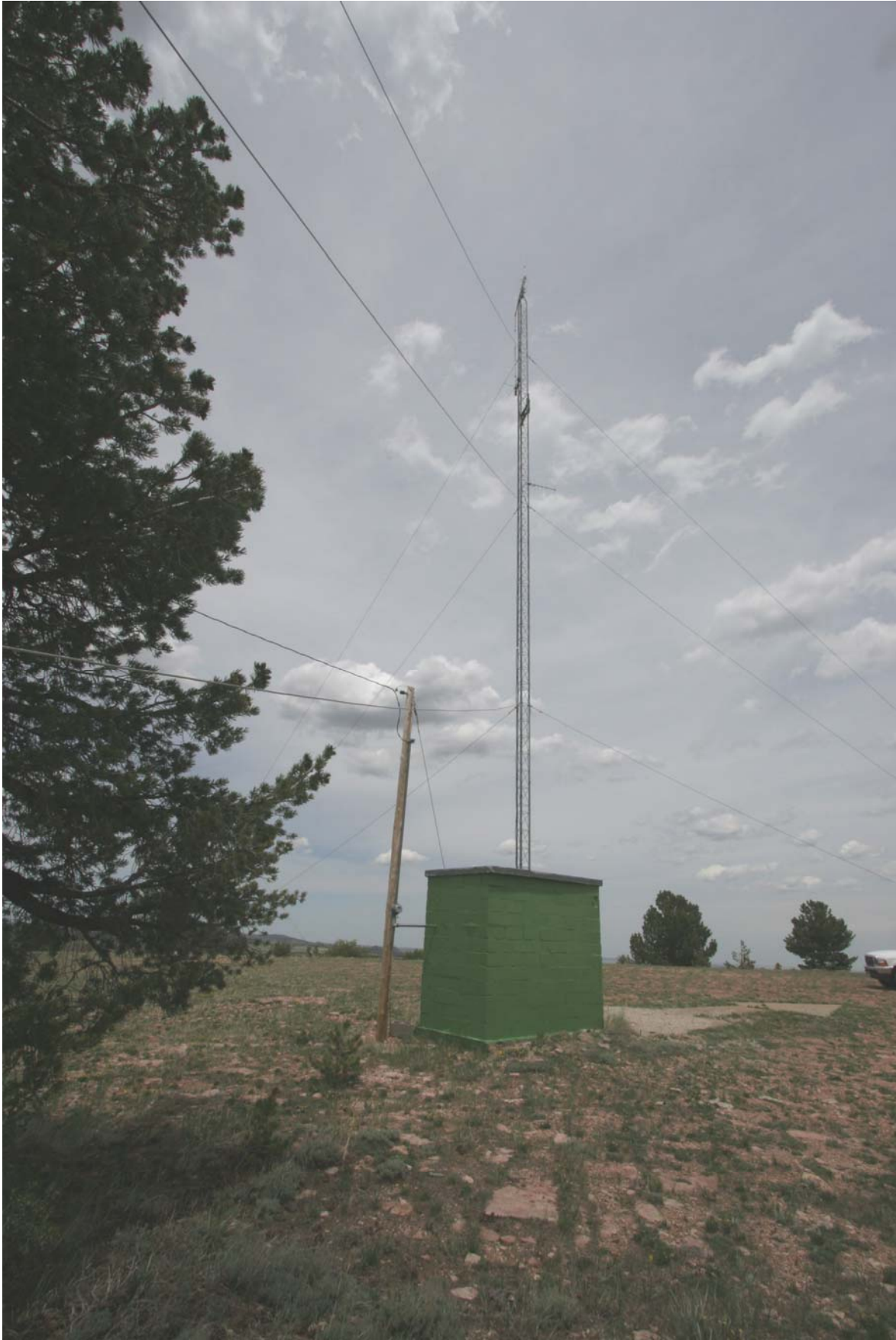
Repeater building, tower and electrical service view looking northeast
