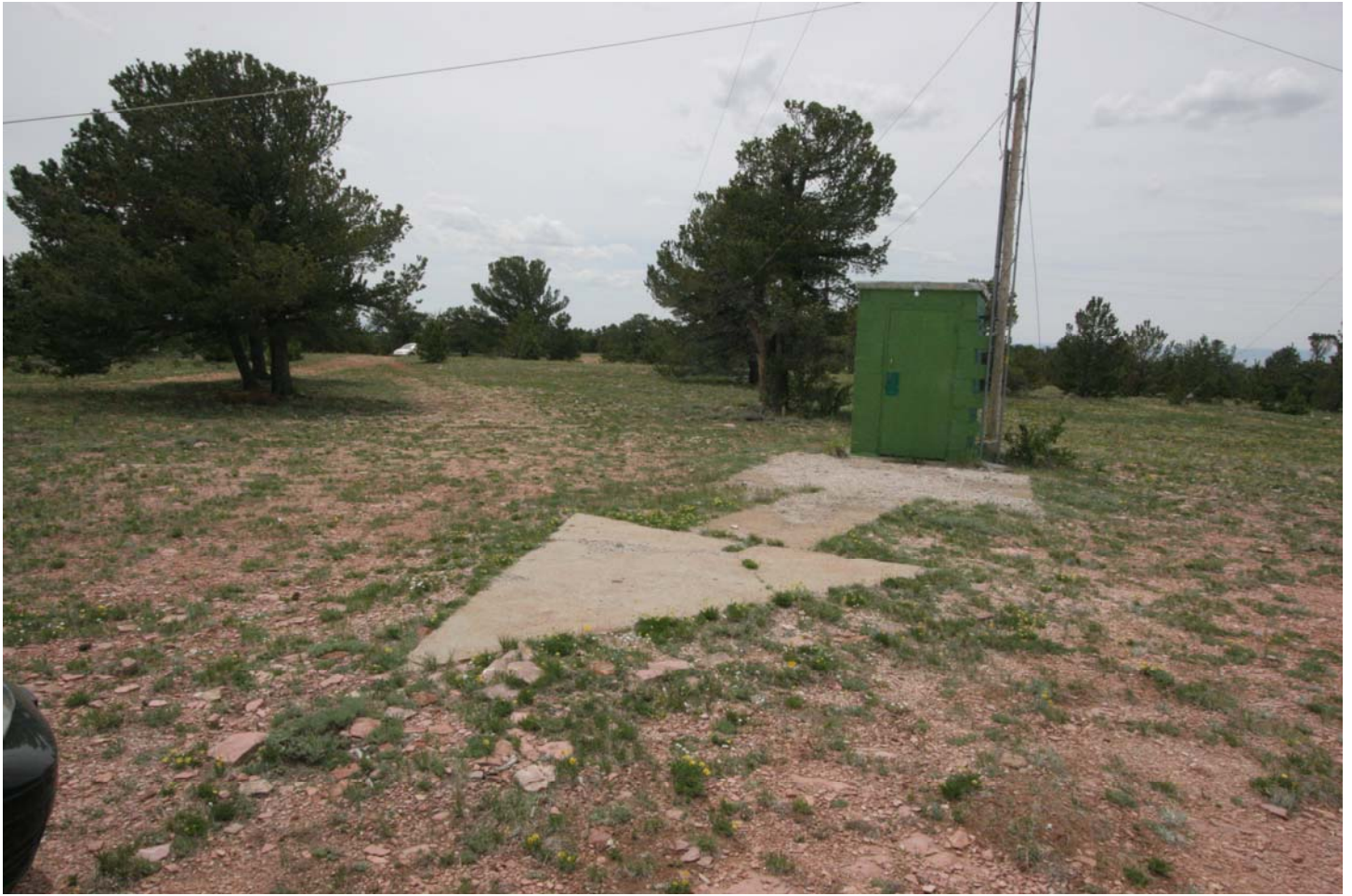
View of the shack looking east. Bill AF7E pointed out the concrete arrow east of the concrete block building was part of an aircraft beacon facility at the site.
