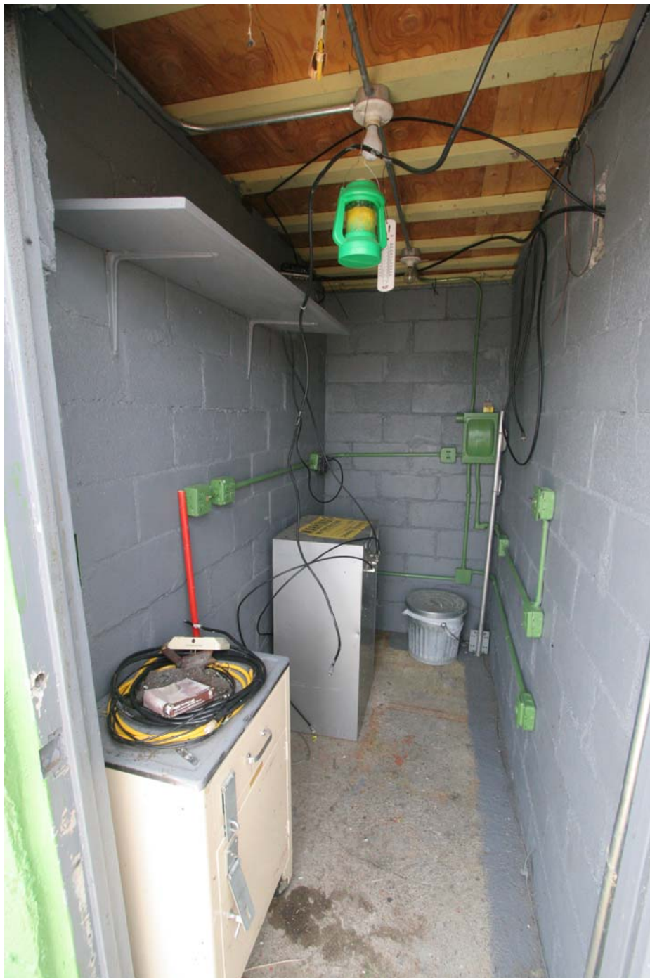
Interior of the repeater .82 shack at Beacon Hill
