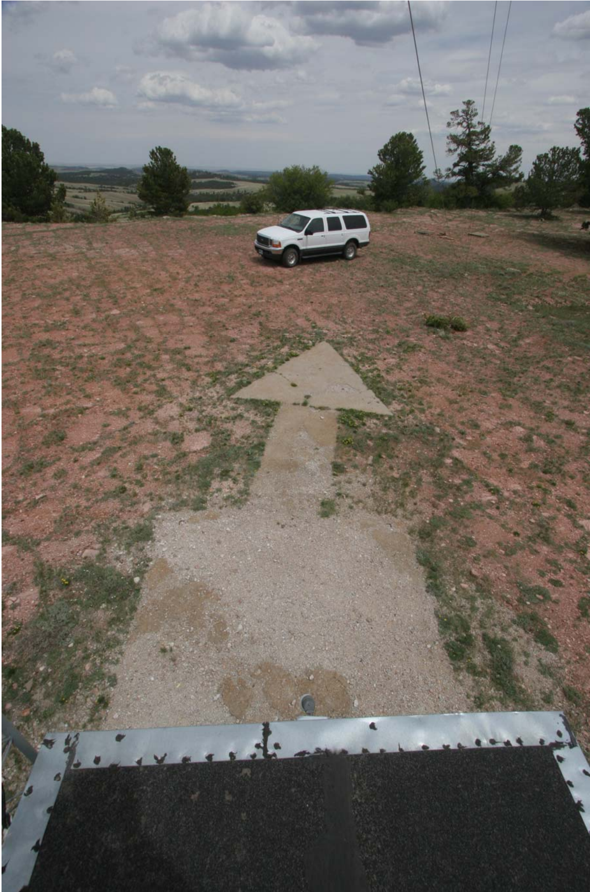
Aircraft beacon arrow from the roof of the repeater building
