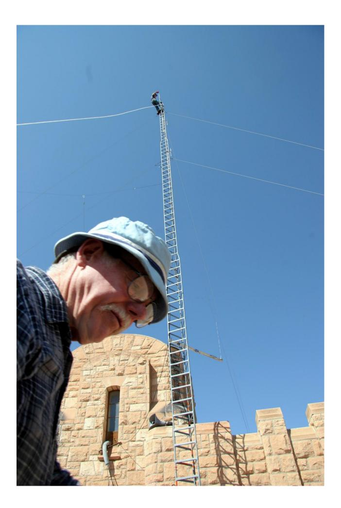
George K7NOI (below) and John KD7NAE (above) install a new 2 meter antenna for the UARC repeater. Thanks to George for donating the new Diamond 7/8 wave vertical antenna.
