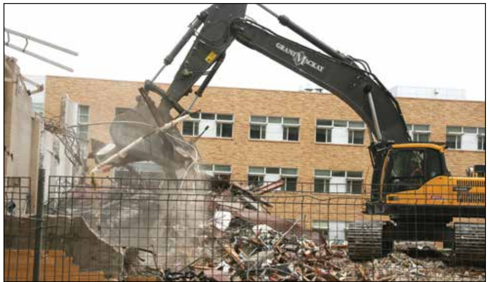
Crews demolish the buildings behind the College of Agriculture Building.
