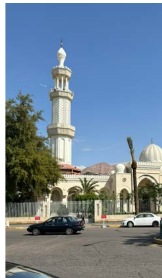
A mosque in Aqaba, a city in southern Jordan.
