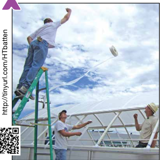
Figure 40. Throwing batten tape over structure for attachment between ribs.
