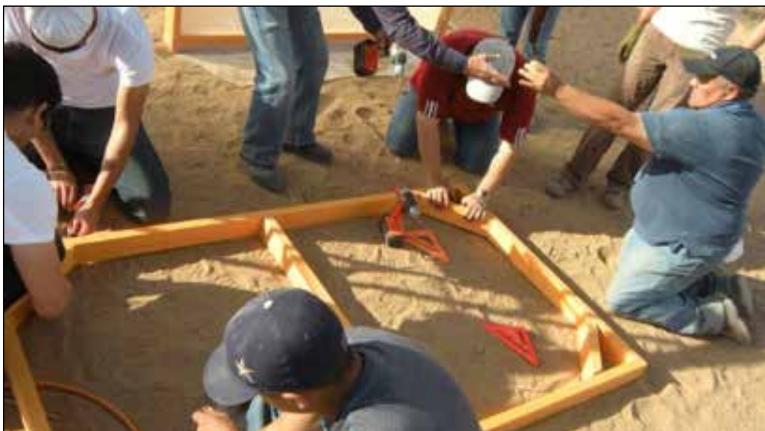
Figure 37. Door Assembly.
