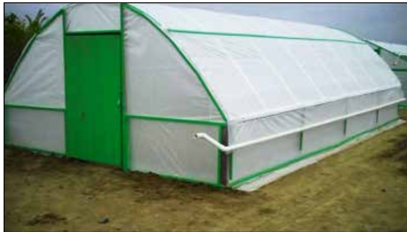
Figure 1. Completed 16' X 32' Hard-sided high tunnel.
