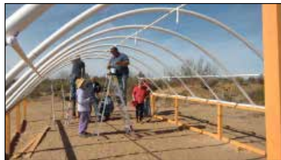
Figure 34. Irrigation purlins.
