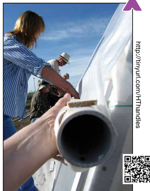
Figure 39. Attaching lath strips to rollup side handle.
