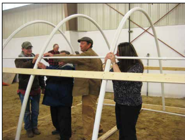
Figure 29. Structural (wooden) and irrigation purlins.
