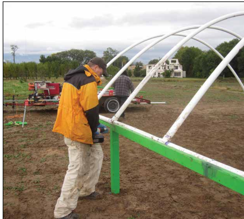
Figure 19. Removing the temporary side rail.
