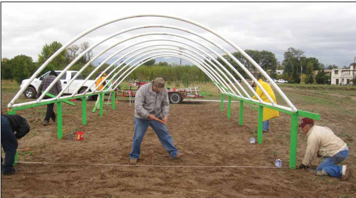
Figure 21. Establishing end wall layout.
