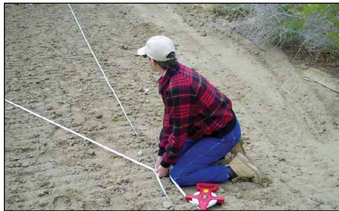
Figure 6. Checking the diagonal measurement of the structure.
