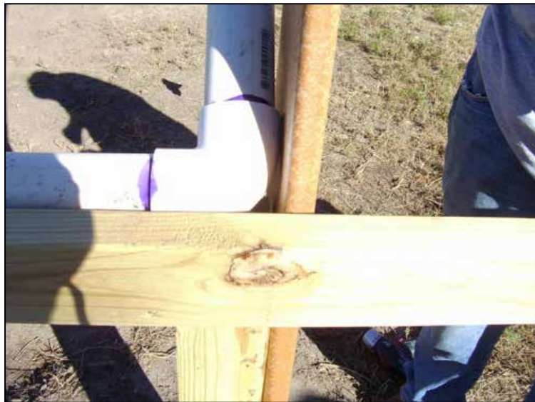
Figure 13. Temporary plate on end of structure to keep first rib assembly flush.
