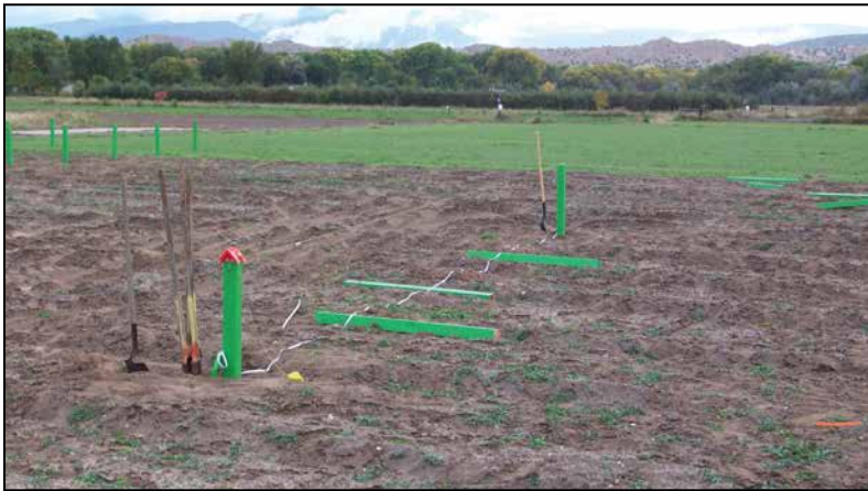
Figure 7. Establishing the Corner Posts.
