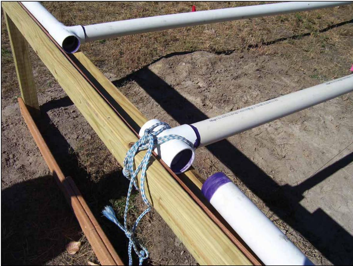
Figure 17. Key Rib prior to installation and attachment to top rail.
