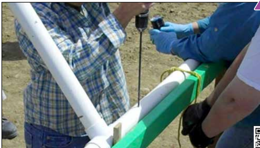
Figure 15. Attachment of Rib assembly to wooden base. Drilling hole for carriage bolt; note 3/8” lath spacer at joint and holding the rib in place with rope.
