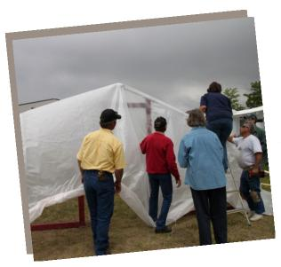
On the ends, stretch the plastic tight over the 2 inch plastic pipe and sandwich the plastic poly covering between the  $\frac{1}{4}$  x 2 inch furring stripping and the pipe using 1 inch screws.
