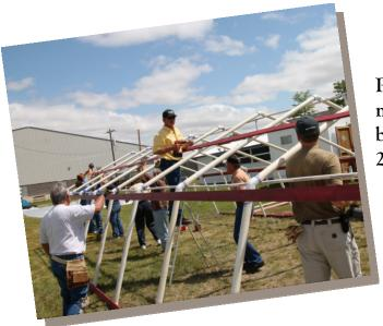
Place another sideboard half way in the middle of the rafters, the length of the building. Secure the bottom side board to a 2 inch plastic pipe.
