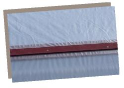
These furring strips can be cut out of a 2 x 4 inch board and driving 1-in. screws every 2 ft. (By using screws in the baseboard, it is easy to remove or replace plastic covering at a later date)
