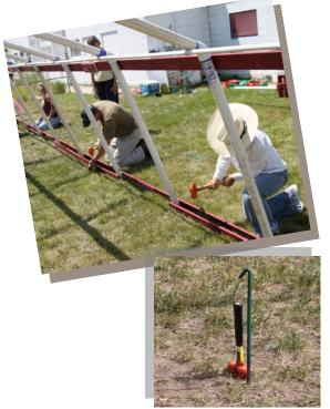
When boards are in place, drive two 24 inch. Rebar stakes bent in a "J" design over each board. This will help keep the hoop house anchored during high velocity windstorms. Repeat process on other side.
