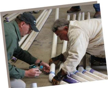
On a flat surface connect two of the 7 ft. 6 in. rafters together using a 2 inch elbow with a 45° curve. This will give you one rib for your straight line cold frame that is made up of 3 elbows of 2 inches, 2 legs 5 foot, and 2 rafters that are 7 foot 6 inches long. After priming and gluing all the pieces together you will have 9 ribs.
