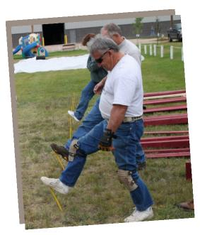
Long both lengths of the Gothic Style High Tunnel Greenhouse and inside the string, drive 24 in. rebar stakes every 4 ft. apart, 12 in. deep, at 30 degree angles, until you reach the desired length.
