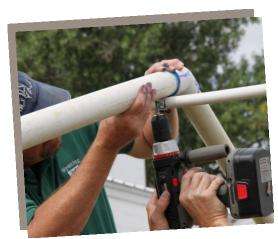
Add 18 inches of ¾ inch PVC pipe to each side. Mark this pipe every 4 foot part and attach the tubular braces to the top of the structure using conduit clamps. Cut off
