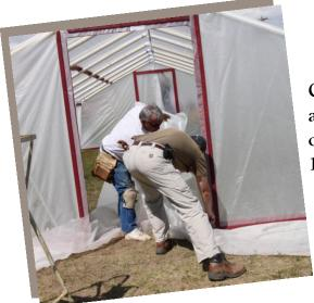
Cut the plastic out of the door frame and set aside until making the door. On the bottom of the hoop house cut all excess plastic to 1 foot out and remove the rest.
