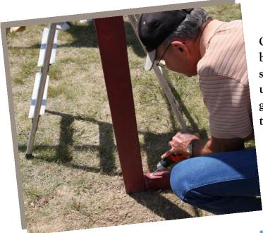
On the ground set a 2inch x 4 inch board from the door frame to the structure. Secure these boards by using 3 inch screws. This board gives support to the hoop house and the plastic will also be attached to it.
