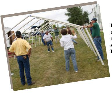
If the rebar stakes are perpendicular to the ground, it is very difficult to place the pipe on the spike. That is why stakes should be placed at a 30-degree angle. Place all 9 ribs on the stakes.
