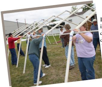
If you are not using the tubular braces for irrigating, you can attach the tubular brace directly to the 2 in. pipe using a 2-in. decking screws. If you will use the tubular brace for watering, you must use a ¾-in. one-hole or two-hole conduit clamp to attach the pipe.
