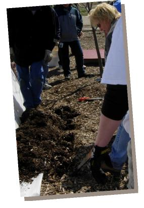
When complete, shovel dirt onto the extra plastic at the base of the hoop house. This will keep wind and the draft from entering the hoop house.
