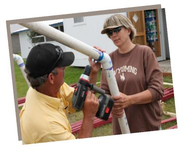
These markings will correspond with the distance between each of the 2 in. ribs. Start attaching the tubular braces from the front of the hoop house. Make sure the brace is flush with the outside of the first rib, and that the markings should coincide with each other. Attach the pipe above the 2 inch 60° elbows.
