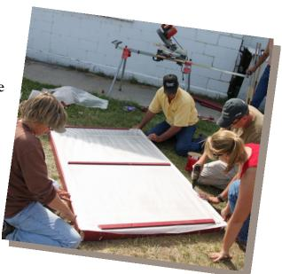
Attach two 3 inch hinges to the side of the door and hang the door in the door frame. On the inside of your hoop house door frame attach 1 inch x 4 inch boards. This will keep air from entering around your door.
