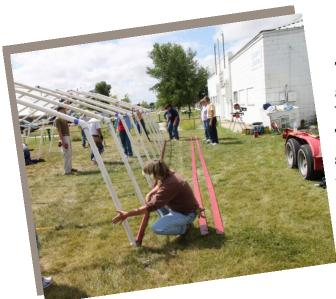
The 10 foot boards are on the outside and the 12 foot board is in the inside. With a brace splice the wood together. There are 3 sideboards per side. Place a side board on the ground at the end of the legs.
