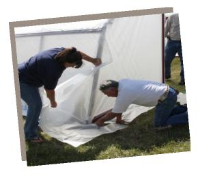
Pulling your plastic covering outward attach the plastic on the bottom to your 2inch x 4 inch boards using furring strips. For the corners tent and cut the plastic in a flag shape. One of the flags will go into the inside and the other flag will be on the outside.
