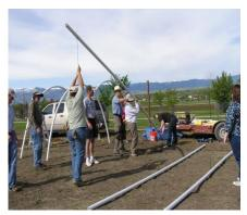
the top end will help to pull and bend the pipe till it can be placed firmly onto the opposite rebar. Make sure all pipes are solid onto the stakes and the ribs are all uniform and even. Adjustments can be made to make them even and line up by using your foot to push in or out on the rebar.
