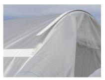
bottom of the door frame up to the PVC on both sides of the doorframe. Measure and attach a piece of lath across top of door frame between the two uprights. Holding the plastic firmly and removing wrinkles, attach the plastic to the door with lath all the way around the door. Now still holding the pleats out firmly, and wrinkle free as possible, fasten plastic down on outside of pipe with a section of uchannel.
