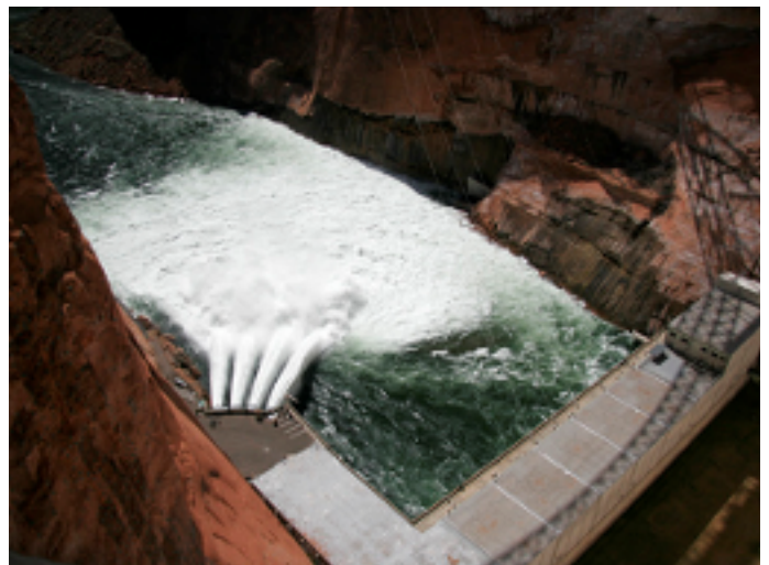
Glen Canyon Dam: All four jet tubes releasing water for high flow experiment. (Photo: United States Bureau of Reclamation)
