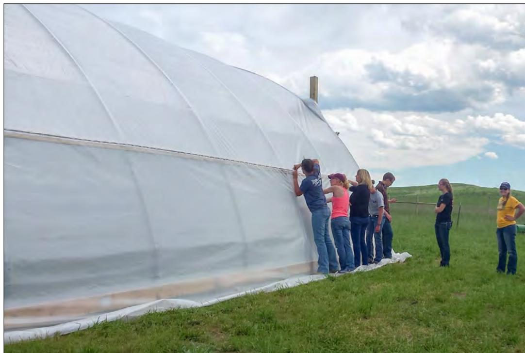
**Figure 2.** The ShREC team installs a cover on one of the two high tunnels.
