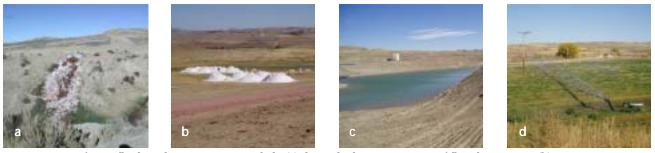
Various options for coalbed methane water use include (a) direct discharge over an outfall rock structure, (b) gypsum treatment, (c) an unlined impoundment reservoir, and (d) land application using side-roll irrigation.
