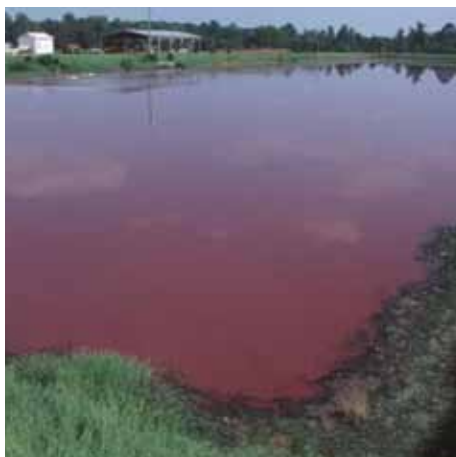
This lagoon captures wastewater runoff.
