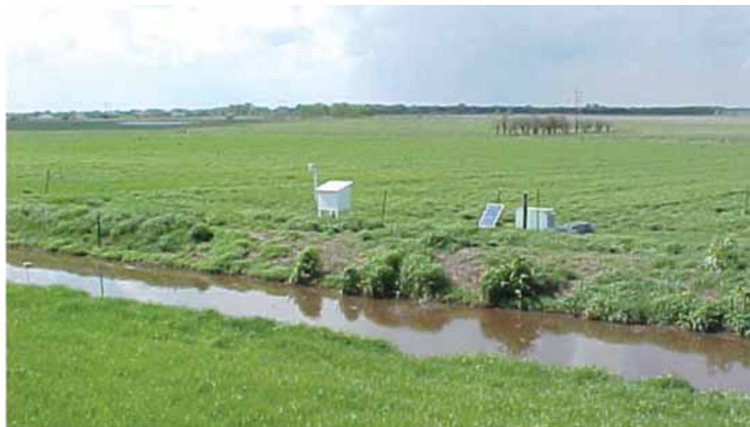
Wastewater is contained in fields planted to perennial grasses or a crop in vegetation treatment systems like this one at the Roman L. Hruska Research Center near Clay Center, Nebraska.
