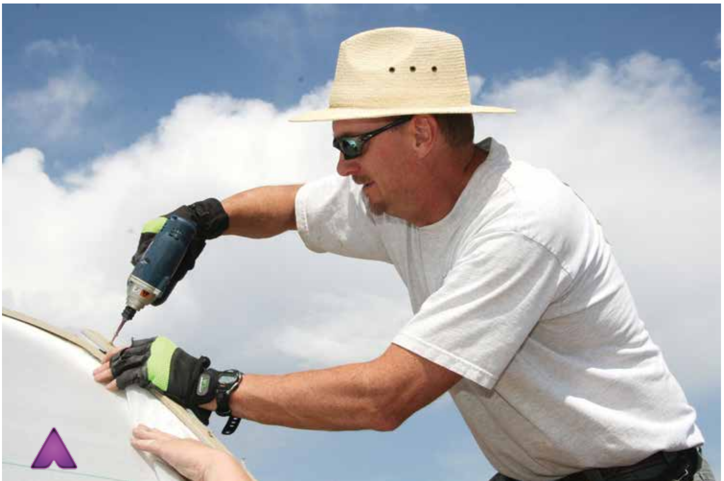
Jeff Edwards, UW Extension educator, ensures a wooden band holding the greenhouse covering will stay in place.
