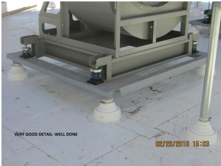
LARGE ROOF FAN FLASHING
