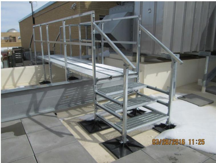
ROOF WALKWAY & STAIR WITH NON-PENETRATING BASES
