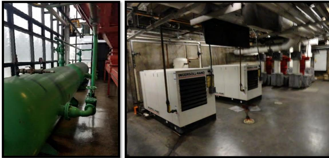
There are many uses around campus for compressed air. These include pneumatically actuated valves/positioners as well as various needs for the boiler system. There are several locations around campus where pneumatic power is generated including the CEP as well as Engineering Addition. New compressors are being installed as part of the new West Campus Satellite Plant.
