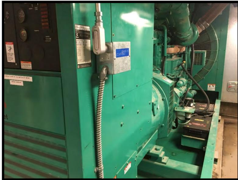
Observations: Most generators have plenty of spare capacity. A centralized system would require significant investment. UW may look to consolidate generators by serving multiple buildings. Systems are often not properly separated into NEC 700, 701 and 702 systems, even with the newer installations.
