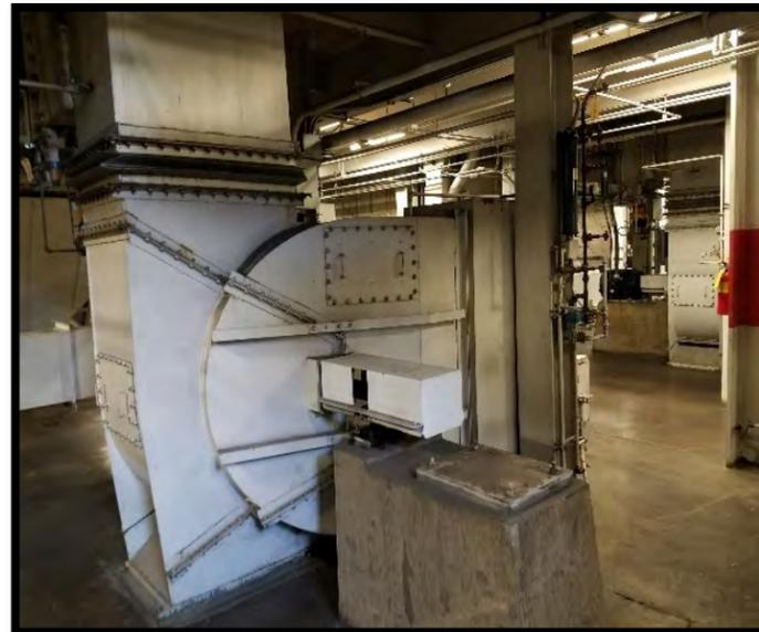
ID Fan: 150 HP, 1192 RPM, VFD present. South ID fan: VFD does work. Harmonic Guard Power conditioning is suspect. Center ID fan: Clarage Fan, manufactured by Air Systems, Kalamazoo, MI. Serial No. 2696CM-5. Size 132, type XLR, series 1250. 1200 Max safe RPM at 430°F.
