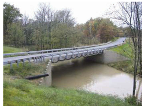
Completed Bowman Bridge, Defiance County, OH
