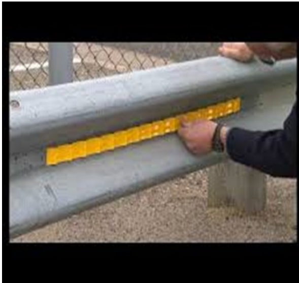
LDS Panel on Guardrail
