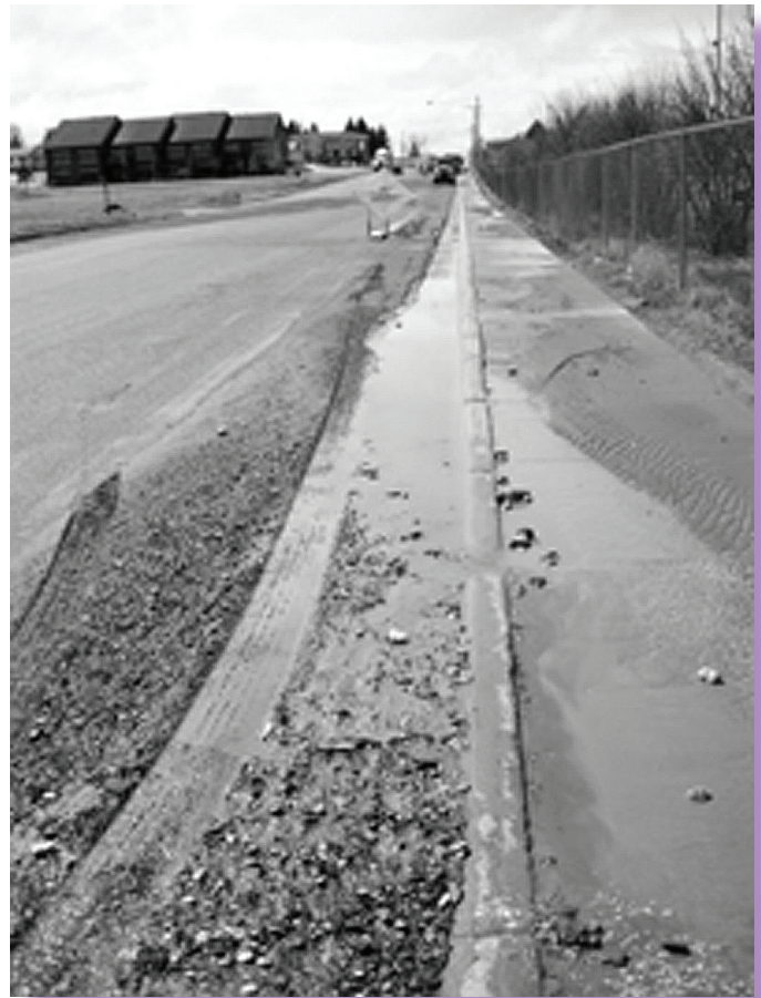
Sediment from urban construction can plug up existing drainage structures such as storm drains and culverts.
