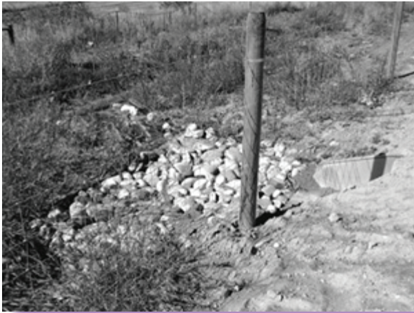
Culvert outlet stabilized with geotextile and riprap.
