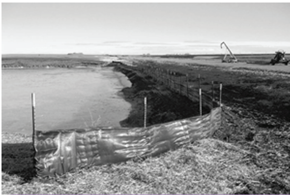
Silt fence used for perimeter control, keeping sediment out of an existing waterway.
