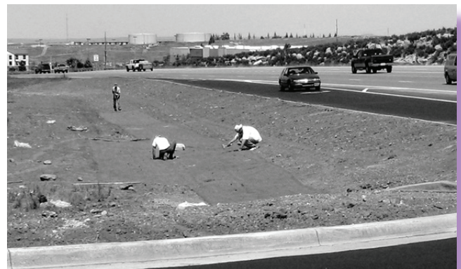
Erosion control blankets reduce erosion until vegetation is reestablished. They also retain moisture so vegetation grows back sooner.
