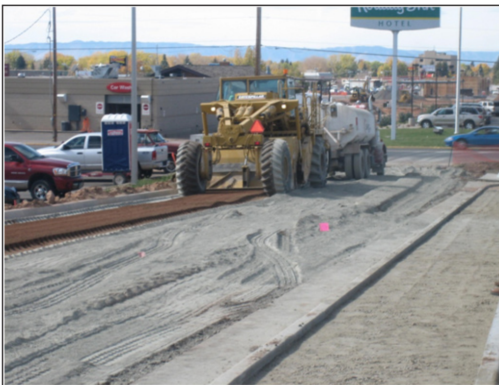
Reclaimer mixing portland cement, asphalt, and base course
