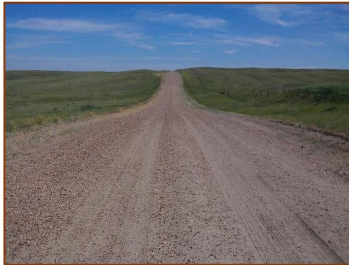
Figure 13 also depicts another real life example of a gravel road. When providing a Level I field evaluation score, this roadway may receive a score of three in the General category, due to the presence of loose aggregate/gravel significantly affecting the safety of the roadway. It may receive a score of nine in each of the other four categories.
