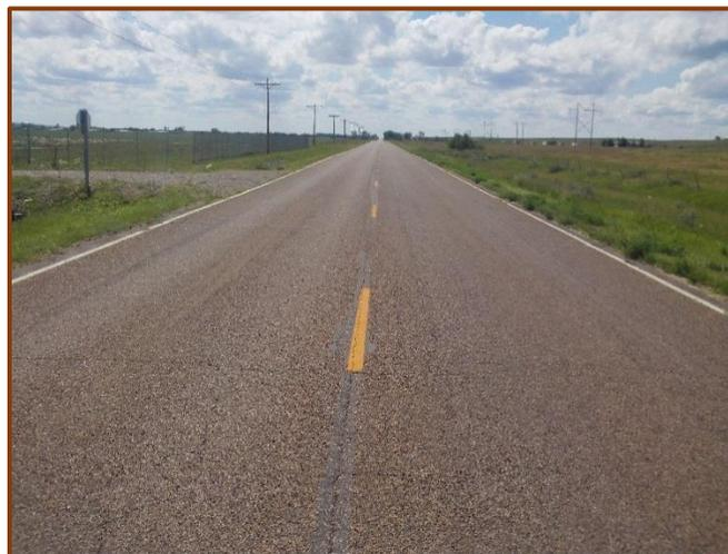
Figure 12 shows an example of a gravel road. When providing a Level I field evaluation score, this roadway may receive a score of seven in the General category, due to the presence of loose aggregate/gravel potentially causing a safety hazard. It may get a score of nine in all other categories.
