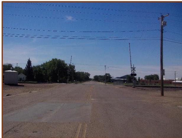
Figure 8 shows another field example of an adequate roadway with minimal shoulder width. Overall, this roadway is in good condition, thus it may receive a score of nine in the General category. This roadway may receive a score of four in the Signage and Pavement Marking category due to the faded pavement markings. It may also receive a score of five in the ROW/Shoulder category as it has a minimal shoulder width.
