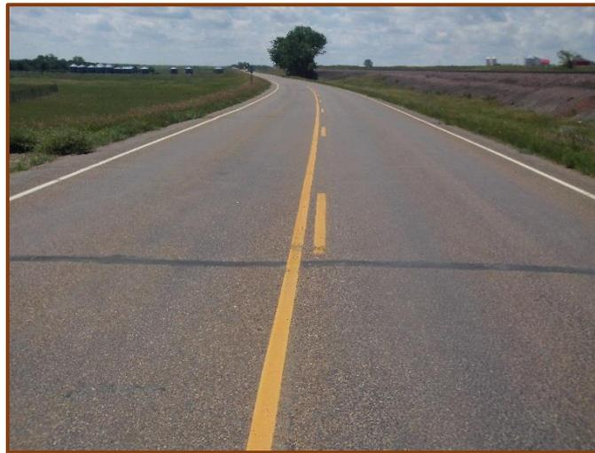
Figure 11 presents another real life example displaying a roadway with a very small shoulder. When providing a Level I field evaluation score, it may receive a score of four in the ROW/Shoulder category due to its width. However, since the roadway seems to be in adequate shape, it may get a score of nine in all other categories.
