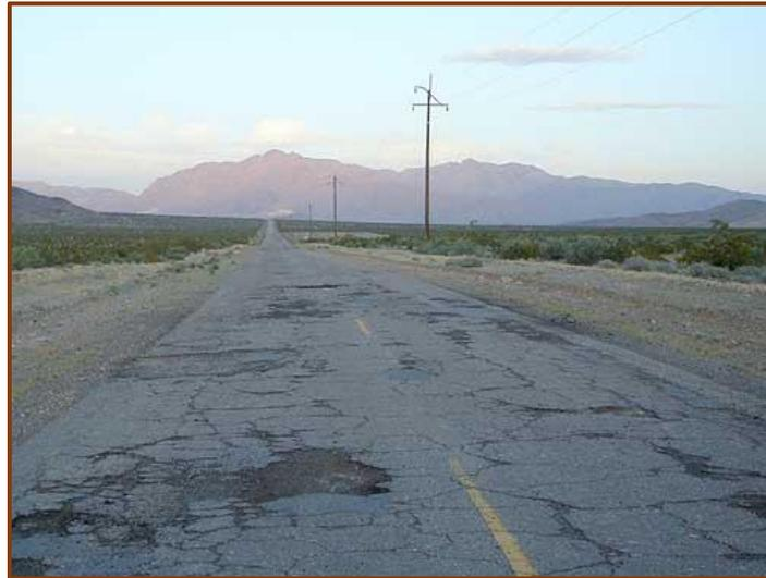
Figure 17 depicts real life example of a gravel road in poor condition. When providing Level I field evaluation, it may receive a score of one in the General category due to gravel defects and ponding or sheet flow areas that could result in safety problems. Nevertheless, it may receive a score of eight or nine in the other categories.
