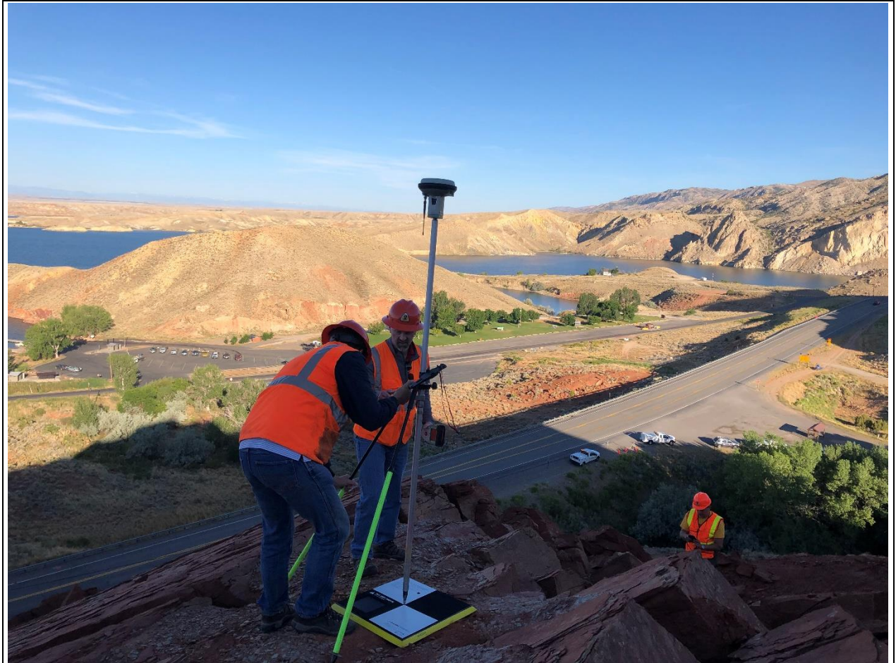
Figure 10: WYDOT survey crew works to verify location of ground control points during photogrammetry project utilizing UAS based data collection.
