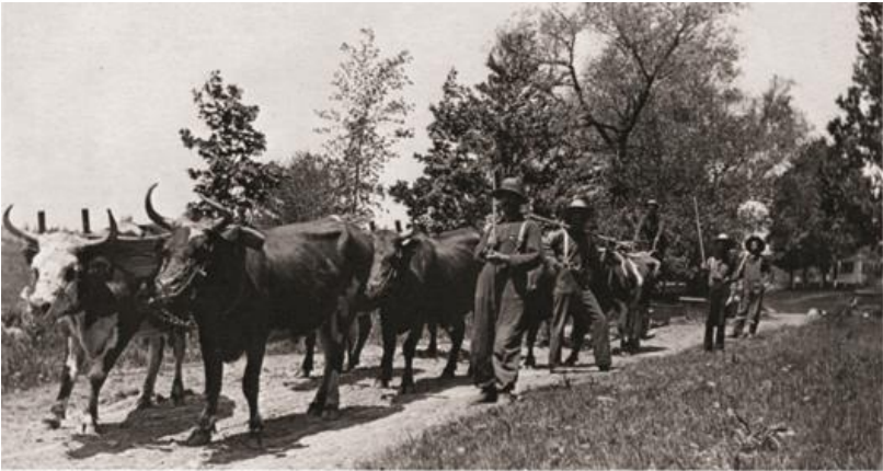
Photograph of an ox-drawn road machine in the vicinity of Plymouth, N.H., circa 1900. The four yoke of oxen attached to this four-wheel grader are indicative of the motive power needed for larger road machines. Such machines had a seat used by a driver when pulled by horses, but required men with goads when pulled by cattle; a man on the machine guided the blade in either case.
