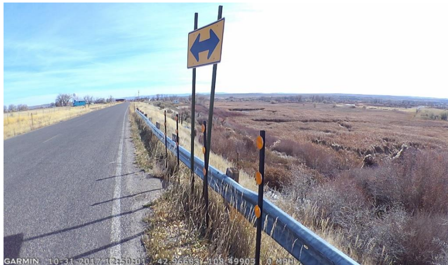
Figure 6. Wrong placement of traffic signs in site No. 1.
