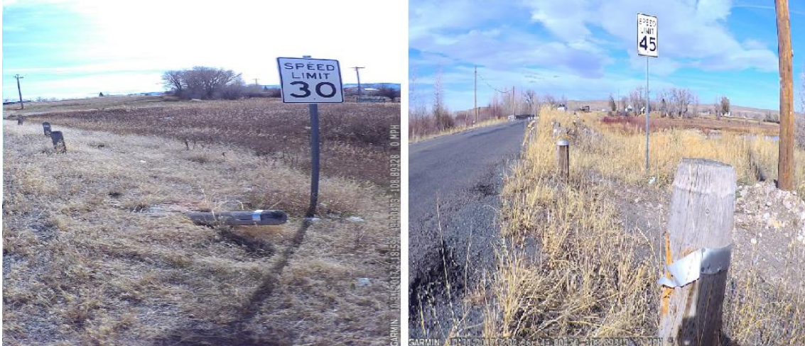
Figure 19. The poor condition of wood-posts at site No. 6
