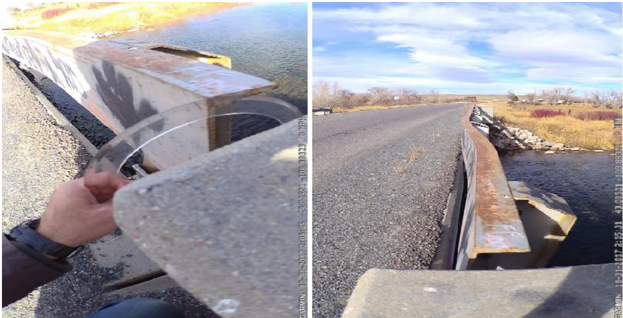
Figure 23. The deflections on the NB of site No. 6.
