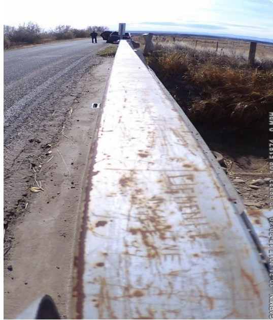
Figure 8. Low-severity deterioration observed in site No. 2.
