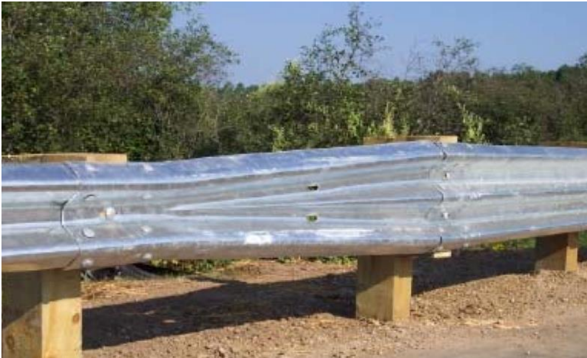
7- Modified Thrie-Beam Guardrail
