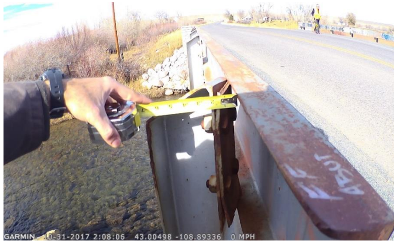
Figure 21. The separated post from guardrail in site No. 6
