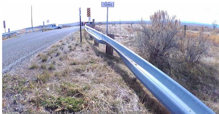
Figure 12. The lower rail cross-section height observed on site No. 3.
