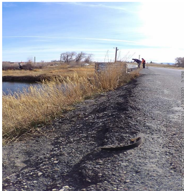
Figure 22. Soil erosion of shoulder site No. 6.
