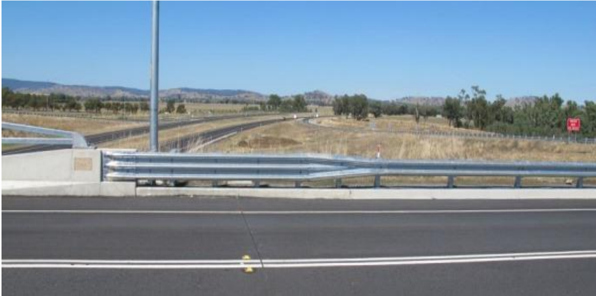
Figure 26. An appropriate design of the bridge transition section.
