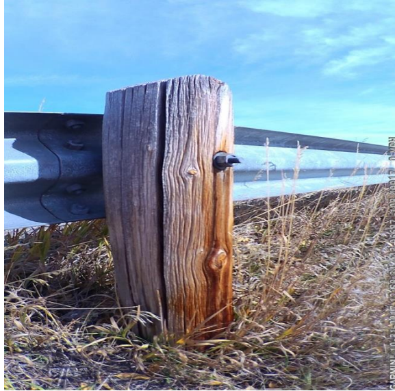
Figure 5. Condition of posts in site No. 1.
